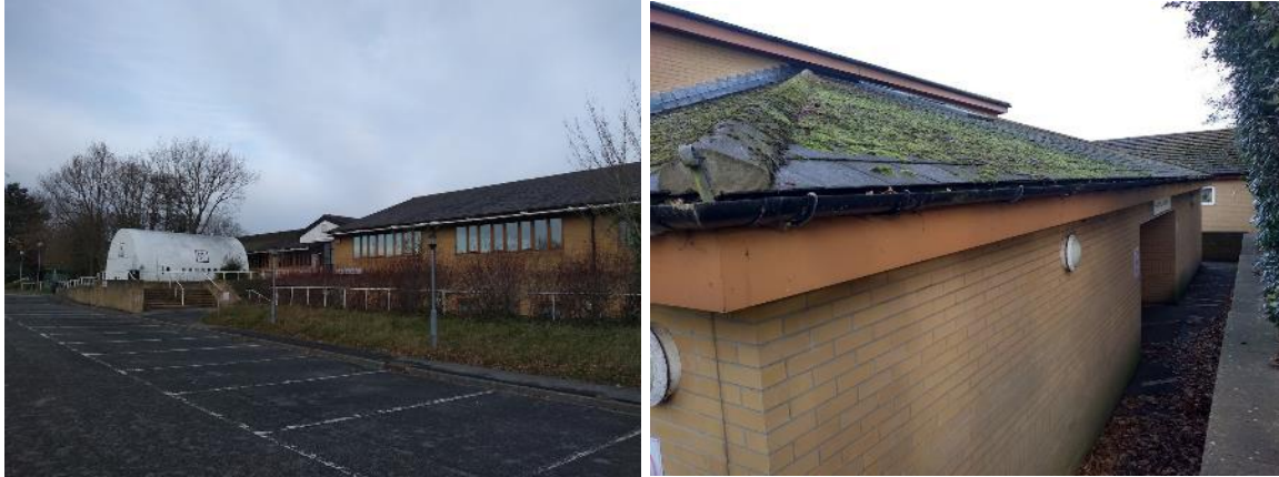
Figure 6 and 7: Main College building
