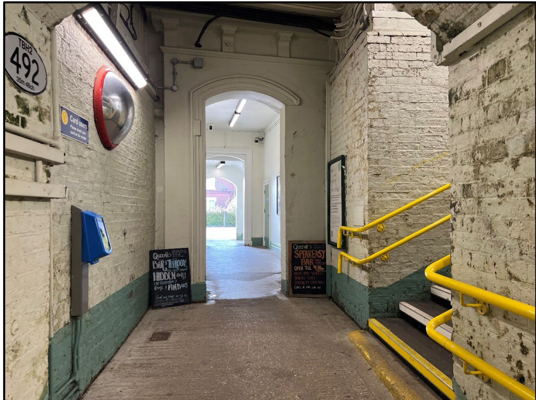
Figure 10: Emsworth Station Underpass
