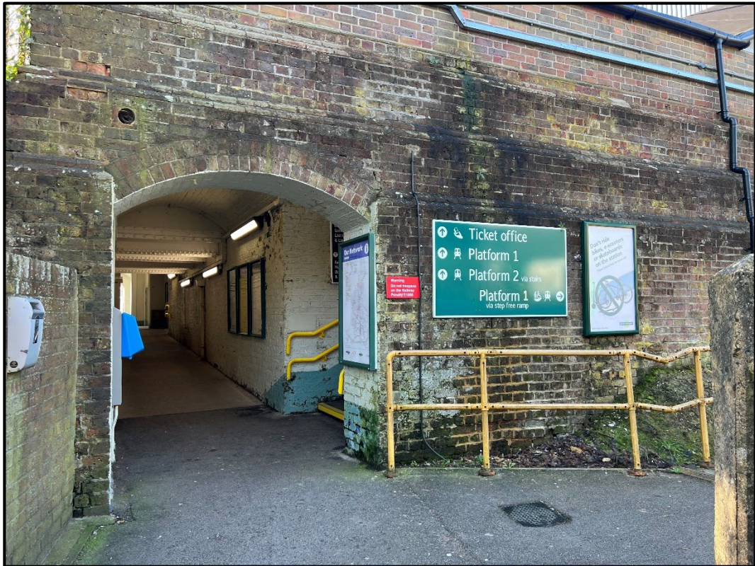
Figure 9: Emsworth Station Underpass
