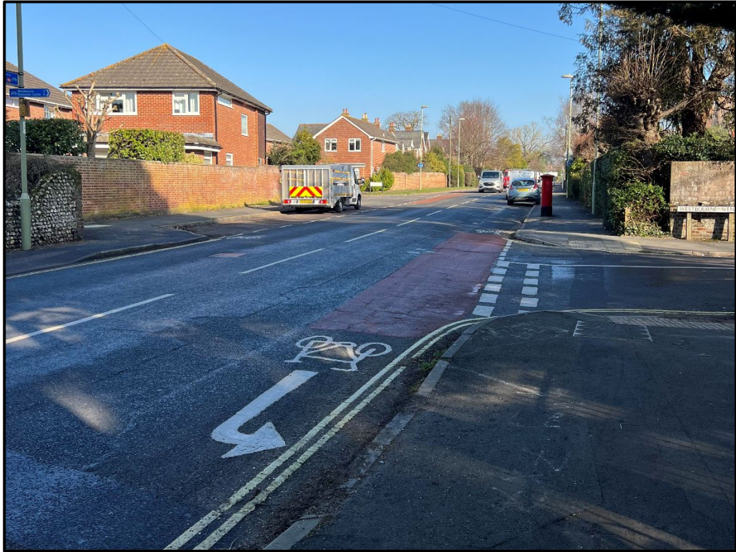
Figure 5: New Brighton Road/Westbourne Avenue Junction
