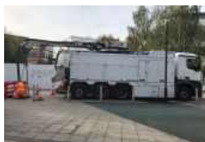
HIGH PRESSURE JETTING
