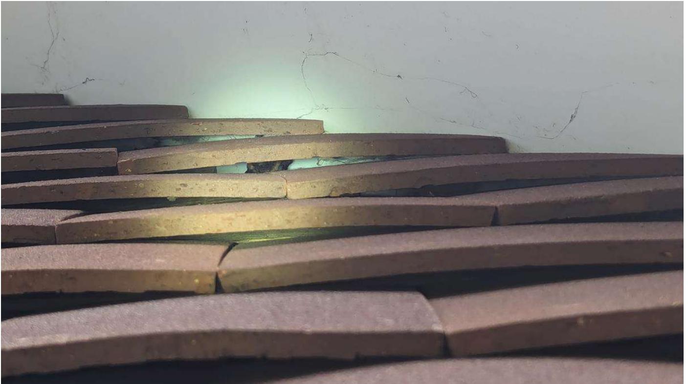
Photo 5 – View of common pipistrelle under hanging tiles.
