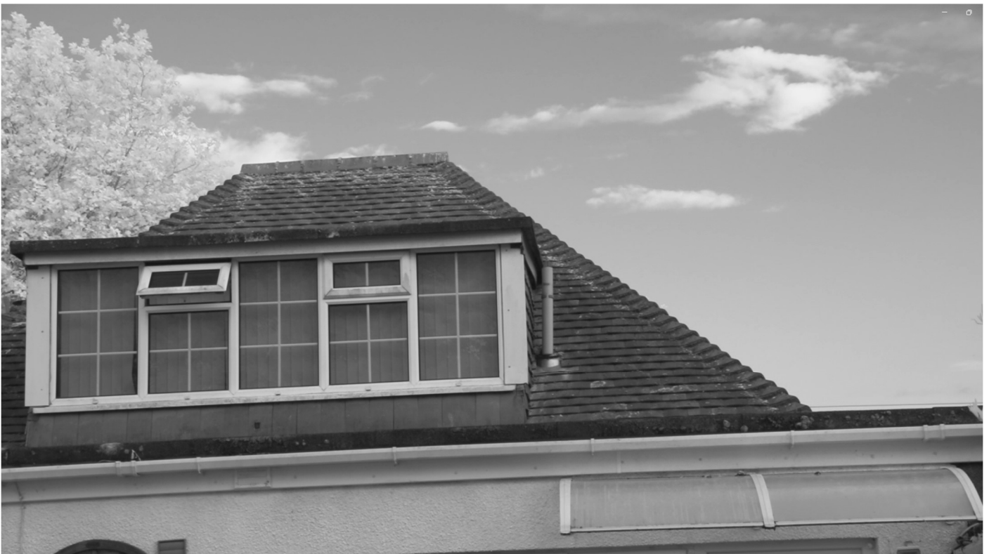
Photo 12 – View of IR3 at start of survey.
