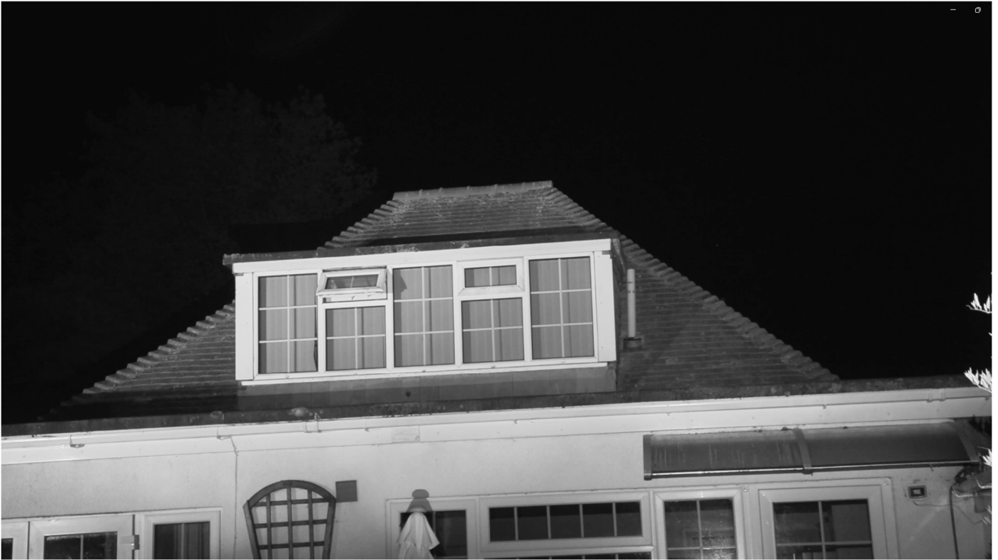
Photo 13 – View of IR3 at end of survey.
