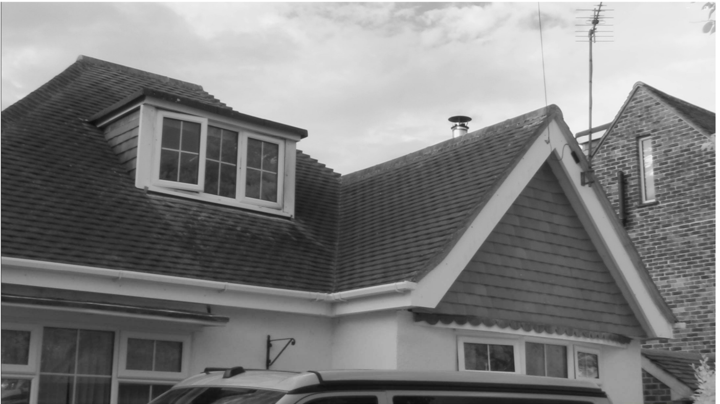
Photo 8 – View of IR1 at start of survey.
