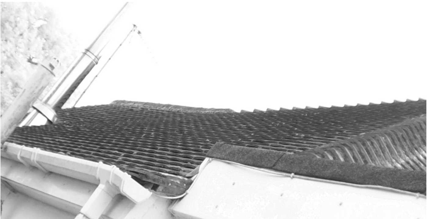
Photo 14 – View of IR4 at start of survey.
