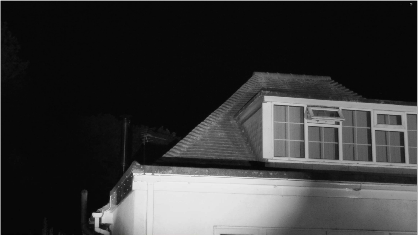
Photo 11 – View of IR2 at end of survey.
