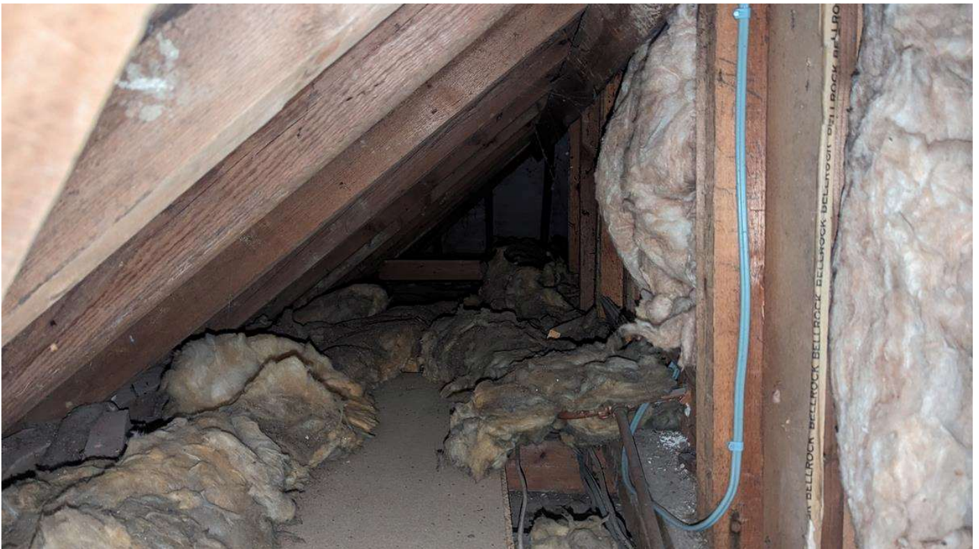
Photo 6 – View inside the loft/skilling space.
