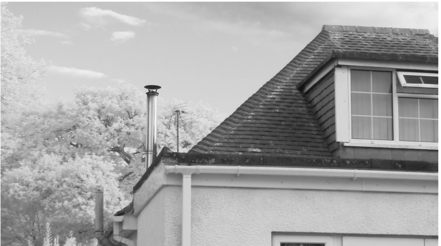
Photo 10 – View of IR2 at start of survey.
