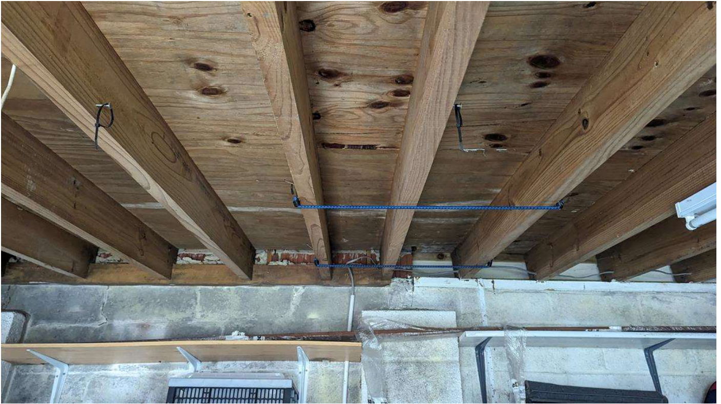
Photo 7 – View inside the garage roof.
