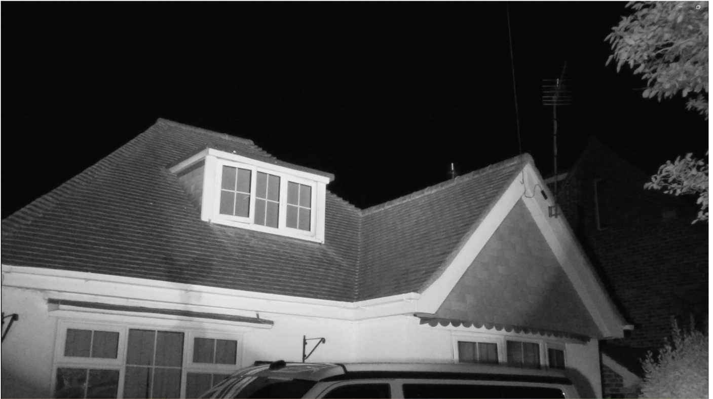
Photo 9 – View of IR1 at end of survey.
