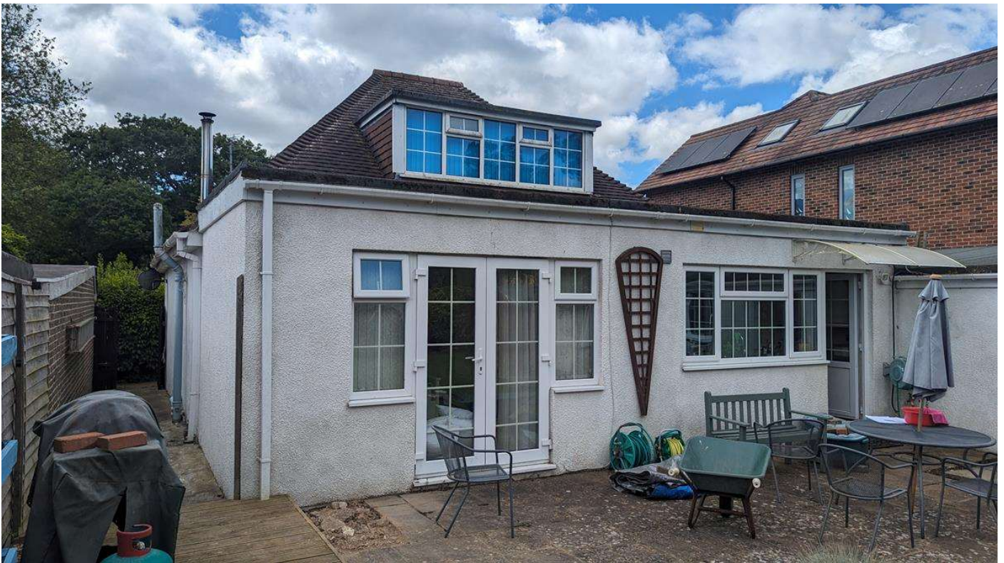
Photo 2 – View of the building from the rear.
