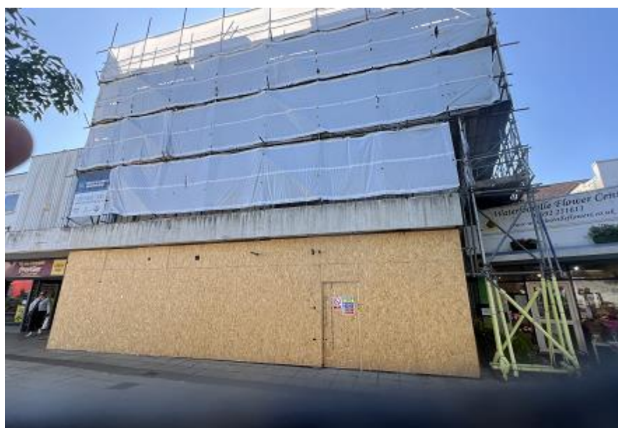
Photograph 5: Nos. 266-268 London Road currently undergoing refurbishment
