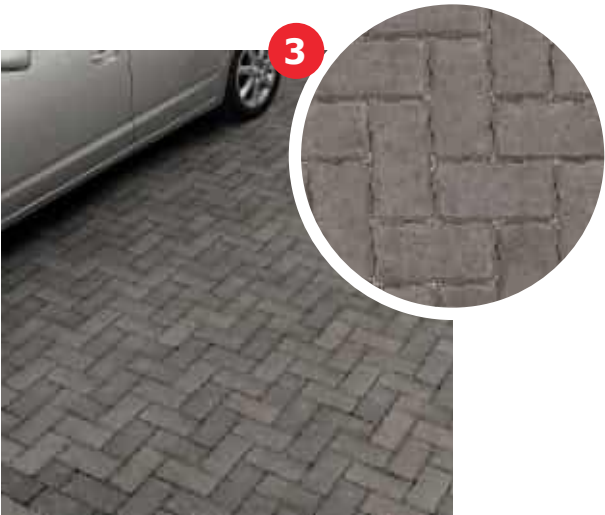
Footpaths: Concrete Block Paving in Charcoal (3)
