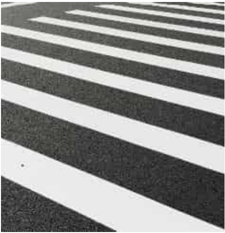
Pedestrian Crossing: Thermoplastic road marking paint in White
