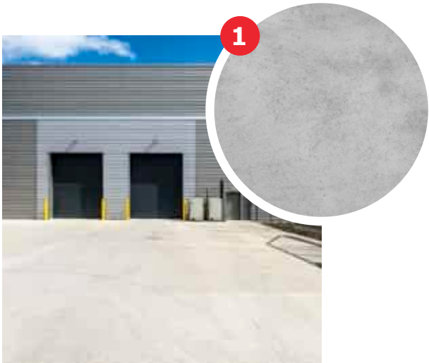
Yard: in Concrete (1)
