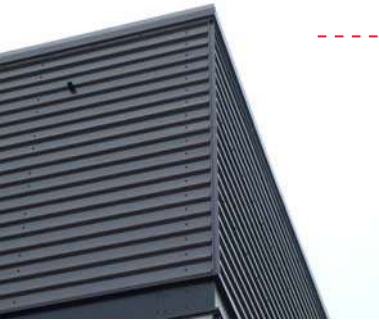
High level cladding: Trapezoidal reverse profile, laid horizontally, Colour: Orion
