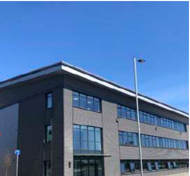
Entrance Curtain Walling
