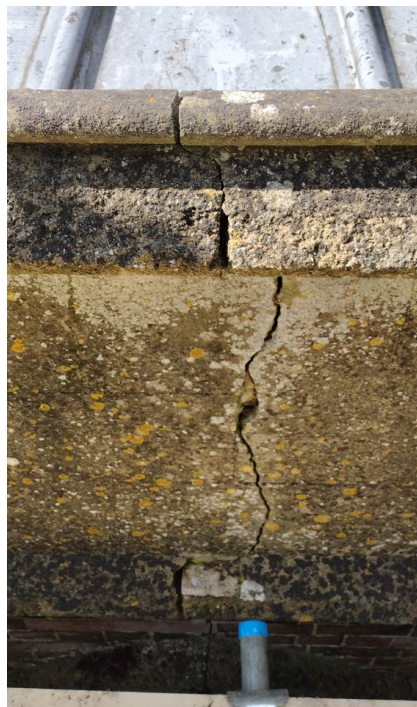
Fig 14 & 15: Image showing significant crack through parapet wall and coping.
