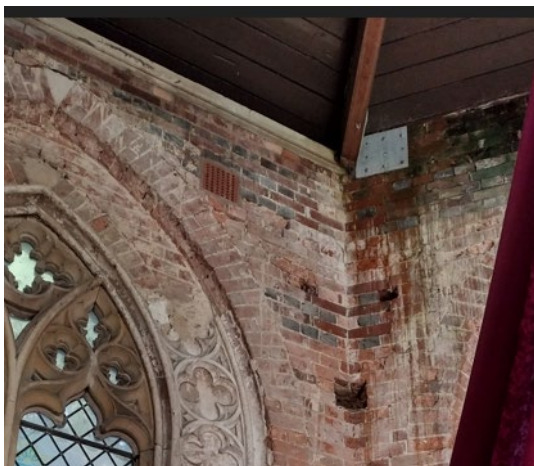
Fig 8 & 9: Image showing damp masonry.
