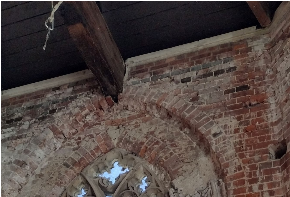
Fig 11: Image showing main roof beam built into external wall
