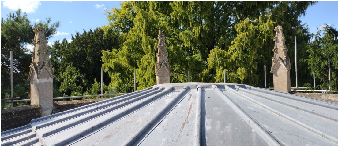
Fig 13: September 2024. Current works commenced, scaffold providing access to roof level.
