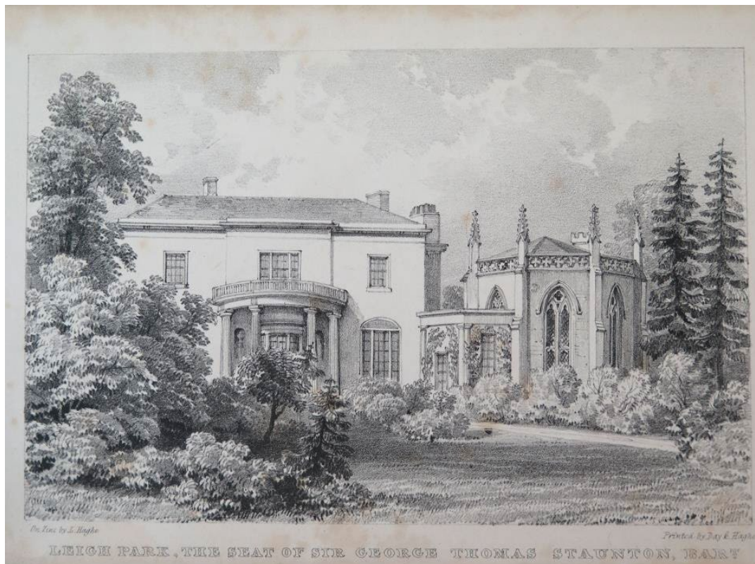
Fig 1: View of Leigh Park House from the frontispiece of “Notices of the Leigh Park Estate” 1836.
