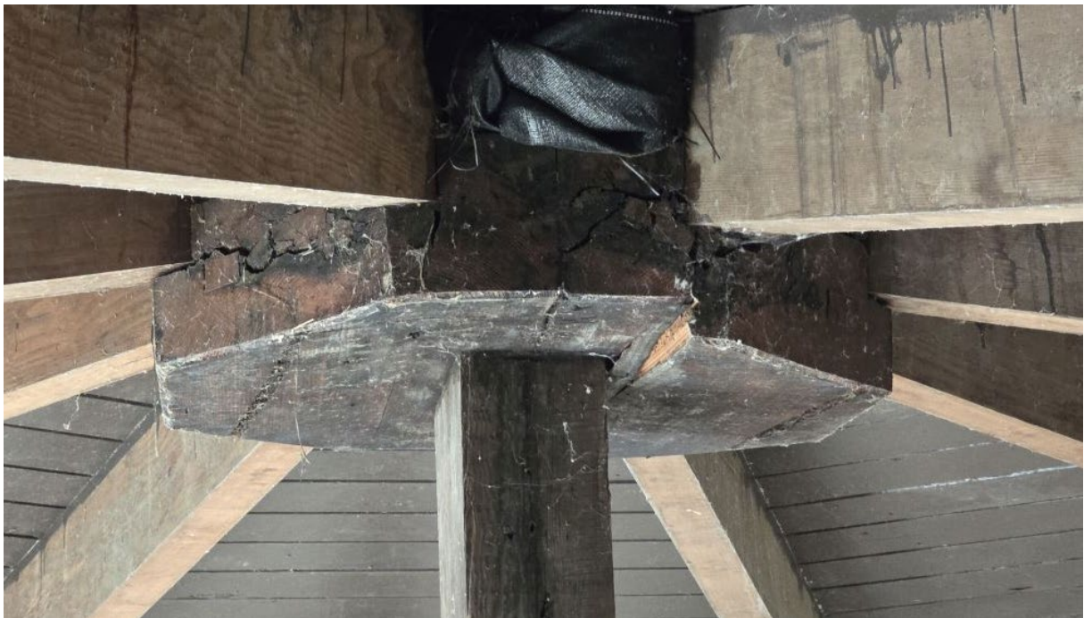
Fig 23: Internal image showing the significant to central octagonal roof plate supporting the hip rafters.
