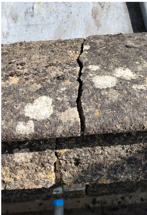
Fig 14 & 15: Image showing significant crack through parapet wall and coping.
