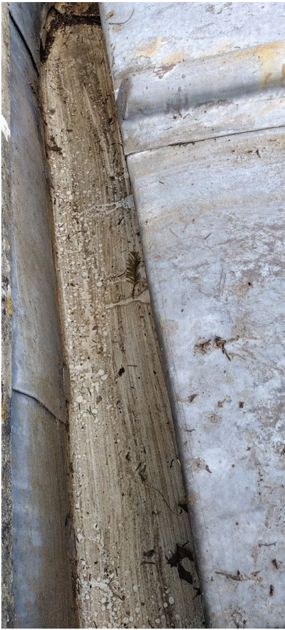
Fig 16 & 17: Image showing cleaned out parapet gutters.
