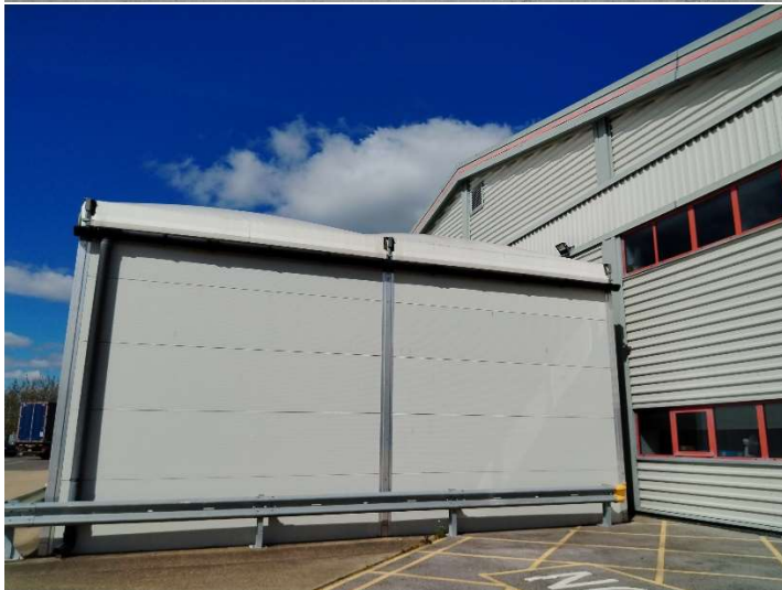
View of principle façade. Note existing colours and textures of the building. Existing temporary covered areas will be replaced with the permanent critical staaina area.
