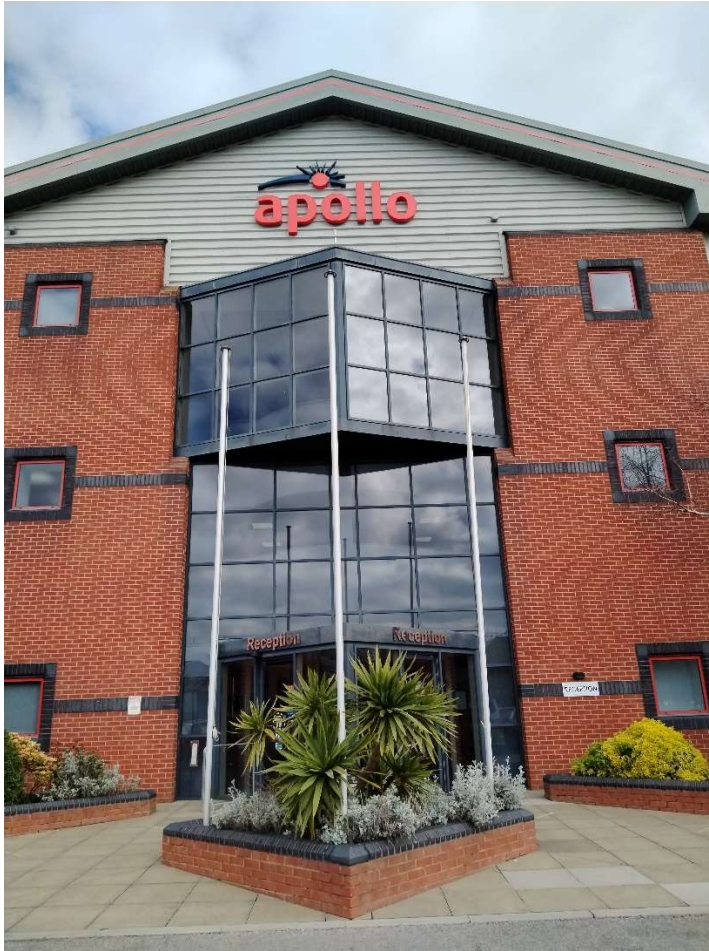
View of principle façade. Note existing colours and textures of the building.
