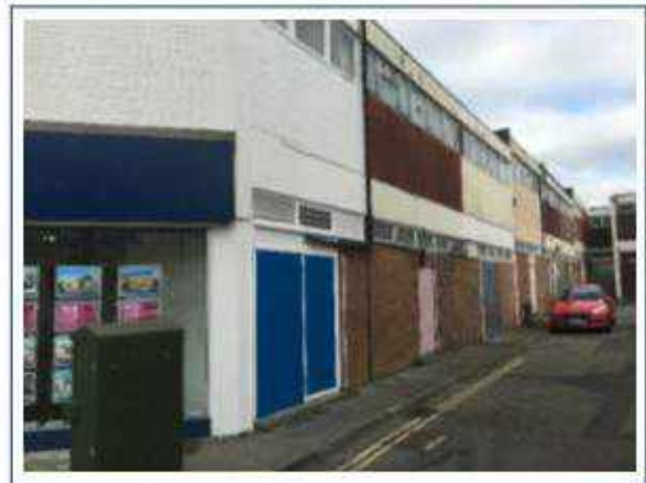
Shared tradesman entrance to the rear of south eastern block
