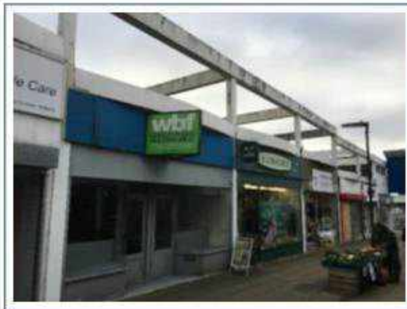
Retail units and view of concrete frame
