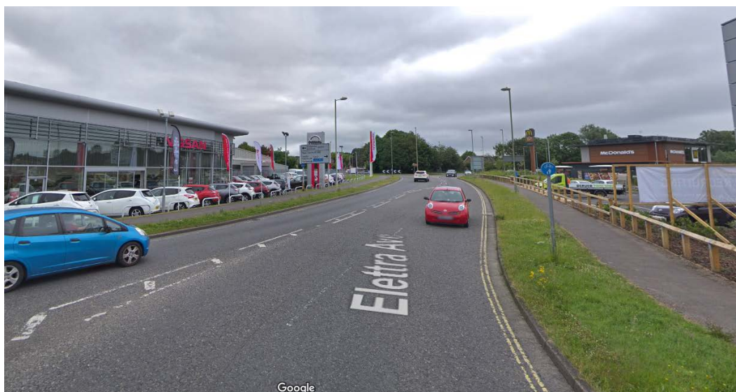
Figure 1 – Footway/Cycleway Along Elettra Avenue
