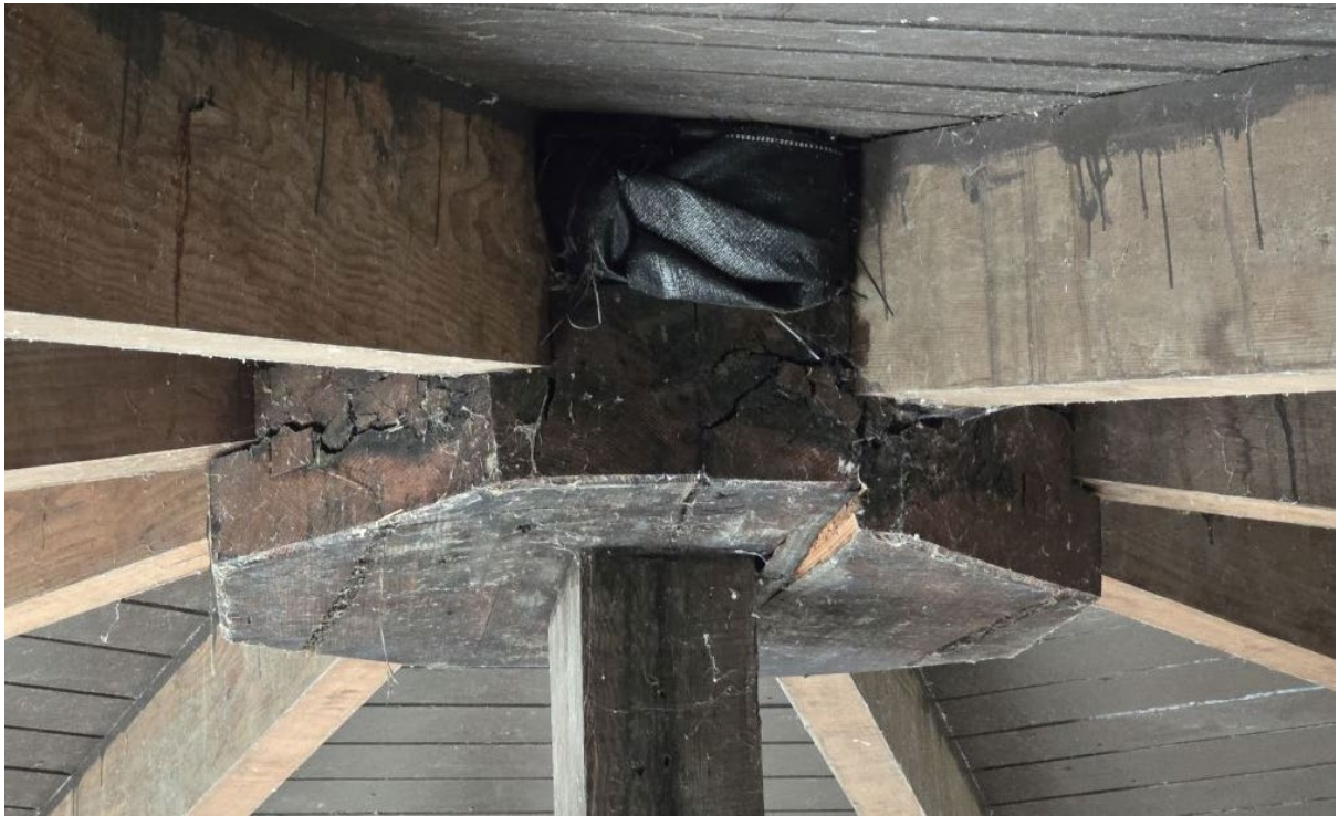
Staunton Farm Gothic Library, Roof Beam Images
