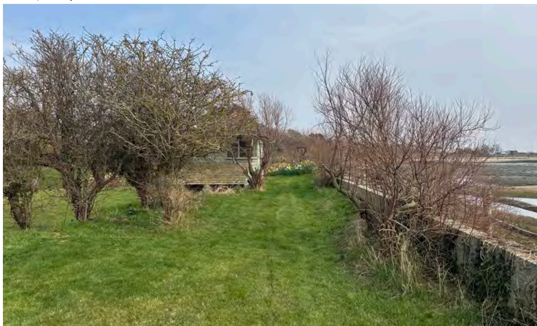
Figure 7. Vegetated garden at the south boundary of the property adjacent retaining wall (taken March, 2025).
