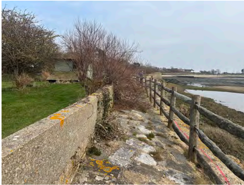
Figure 8. Retaining wall and concrete skirt in main works area with wooden fence bounding walkway (taken March, 2025).
