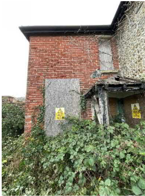
PLATE 27: Eastern elevation of rear "extension"
