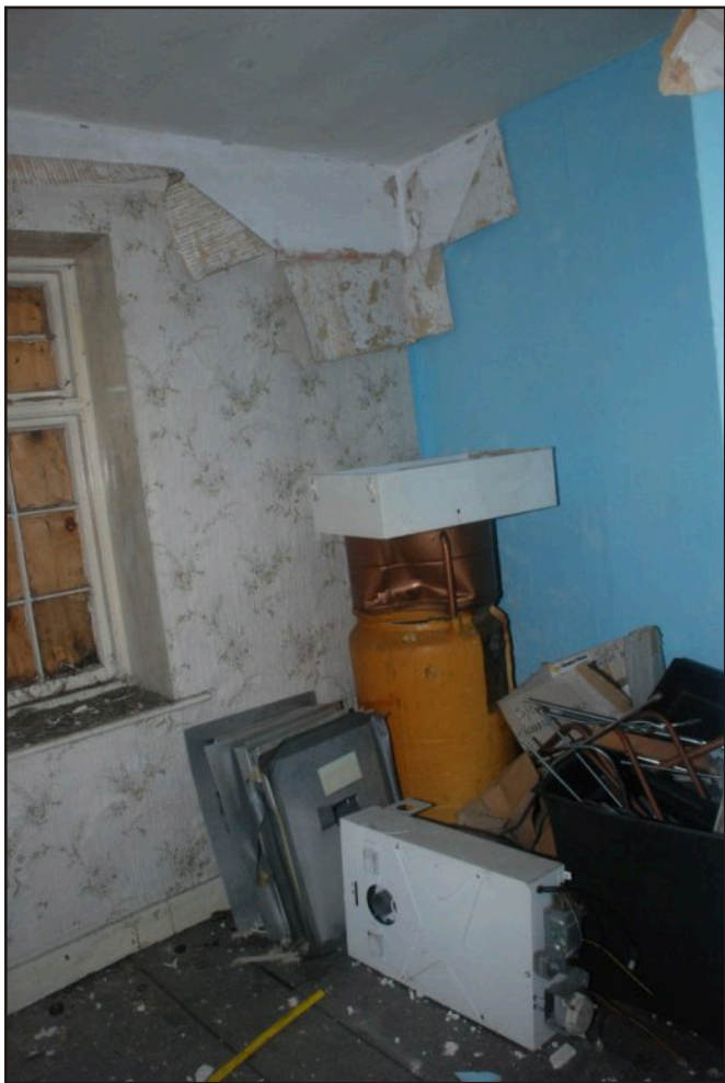
Plate 29. First floor room - note damage to lath and plaster internal walls.
