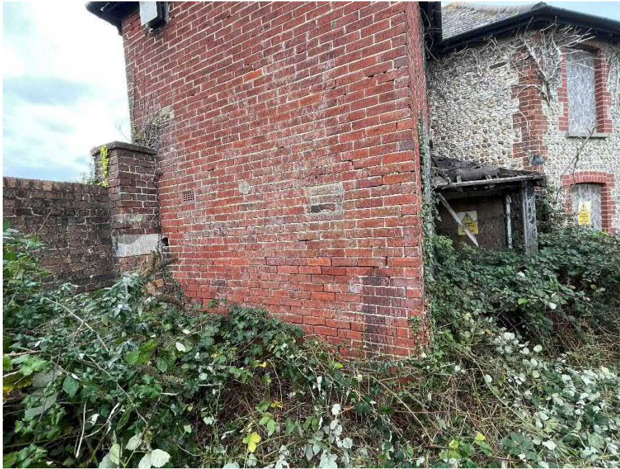
PLATE 23: More detailed view of eastern corner of south elevation of rear “extension”
