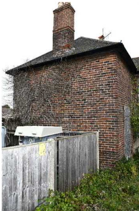
PLATE 4: West elevation of house viewed from south-west
