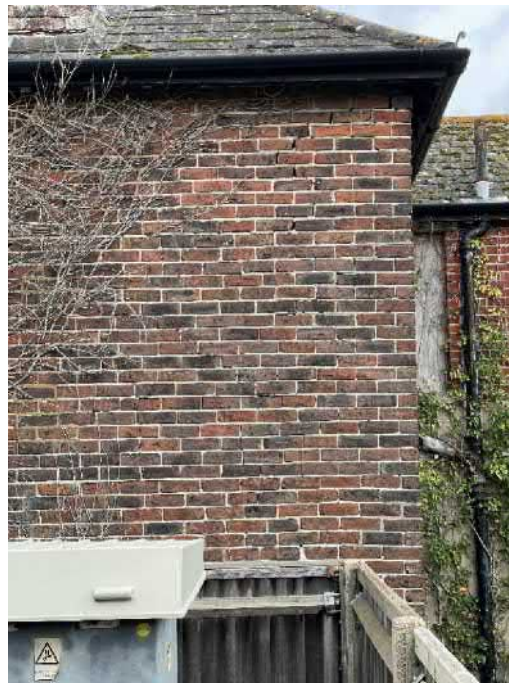
PLATE 12: Closer view of southern end of west elevation in (4) above
