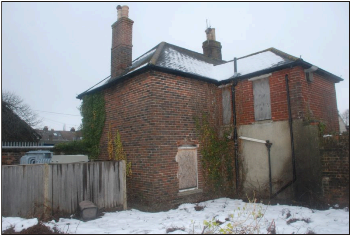
Plate 9. South-west corner of house - note sub-station compound to left of view.
