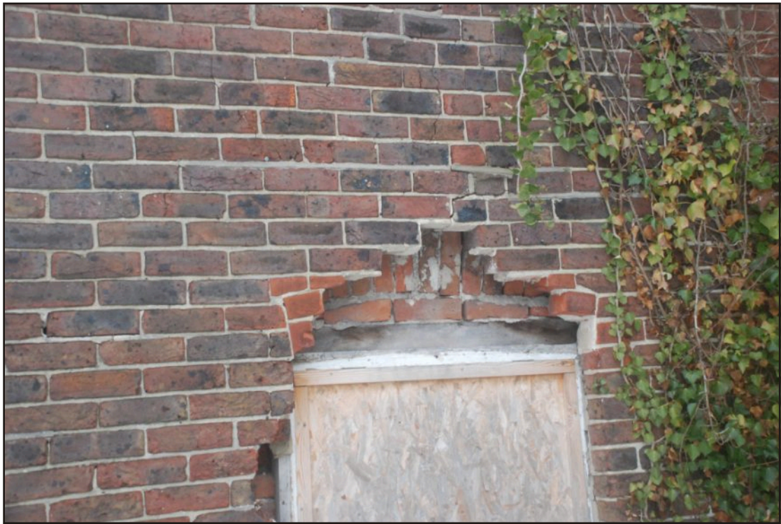
Plate 11. Close-up on (9) above showing failed lintel over ground floor window.
