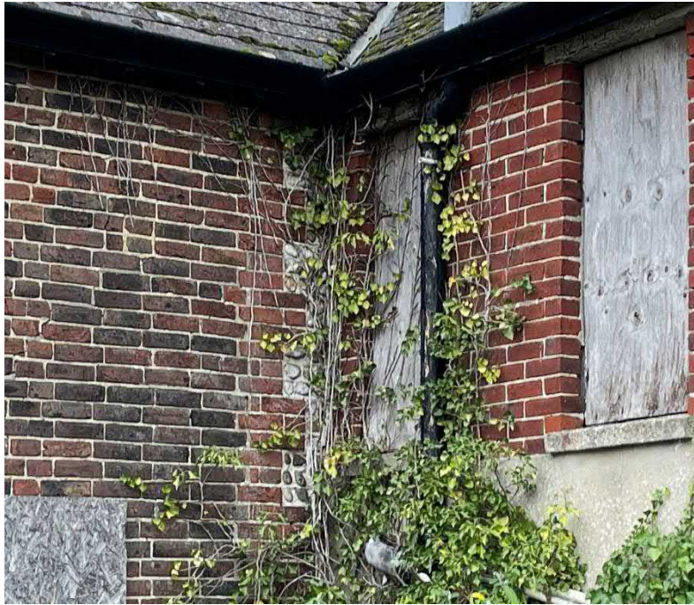
PLATE 19: Detailed view of corner return in (15) above – note change in colour of brickwork where rear extension inserted
