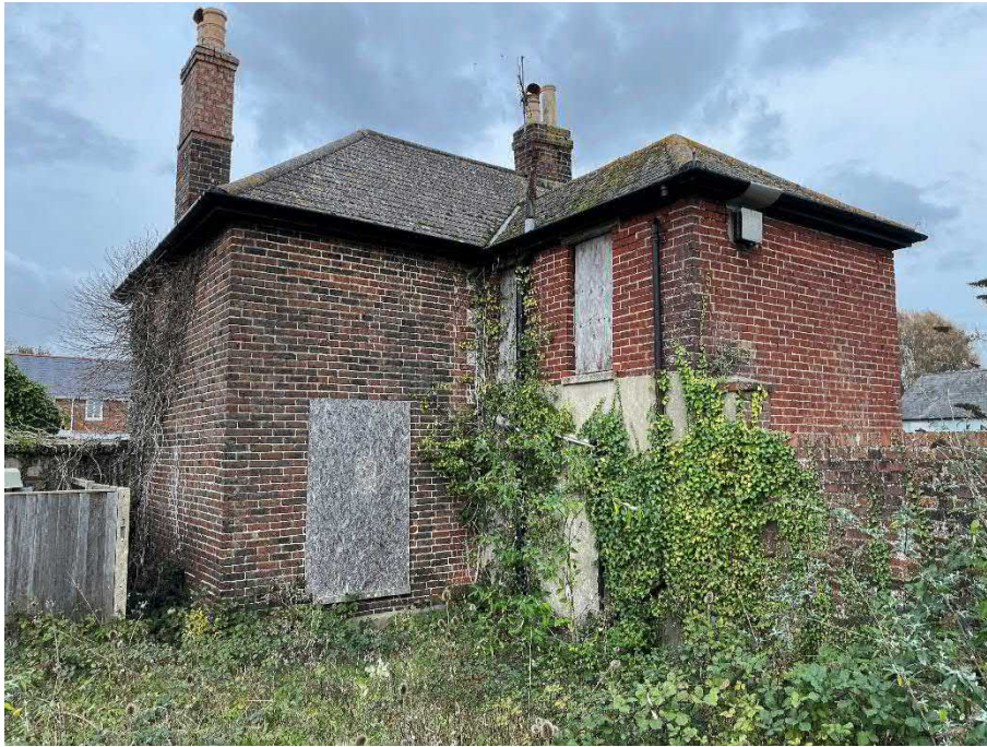
PLATE 5: South elevation of house viewed from south-west with rear "extension" to right of view
