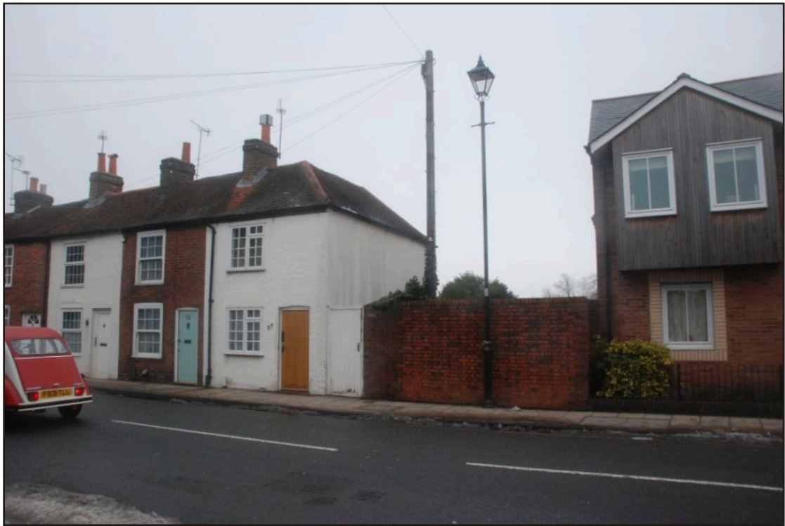
Plate 17. "Access" in (16) above viewed from North Street.
