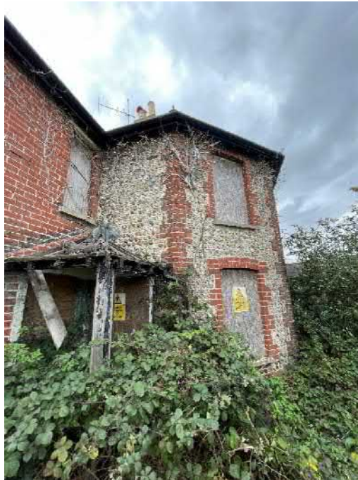
PLATE 7: East elevation of house viewed from south-east with rear “extension” to left of view
