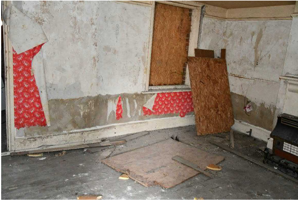
PLATE 45: View on south-west corner of house at ground floor level
