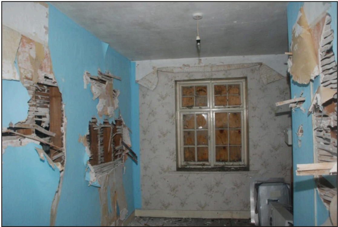
Plate 29. First floor room - note damage to lath and plaster internal walls.
