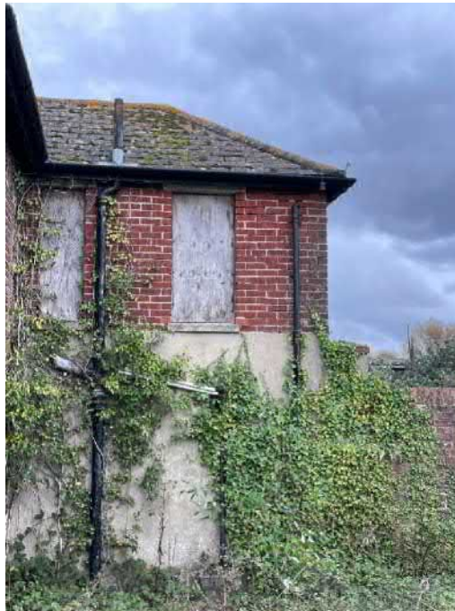
PLATE 20: Western elevation of rear "extension"
