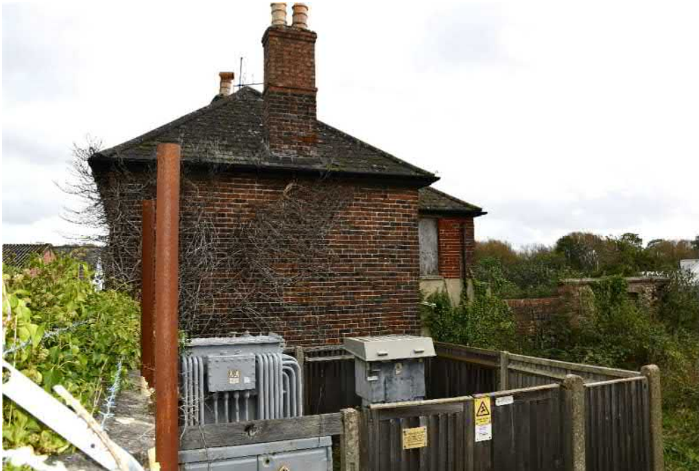
PLATE 3: View on west elevation of house – note substation compound immediately adjacent
