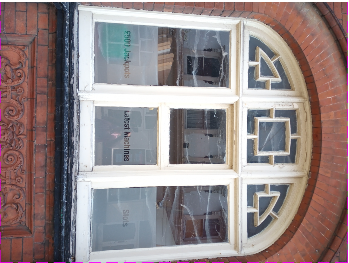
all damaged bricks to be repaired with colour matched resin
