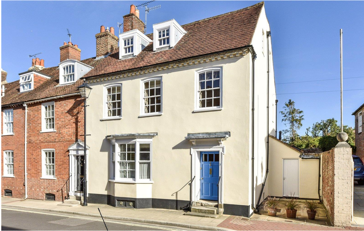
Photograph 1 – North West Elevation
