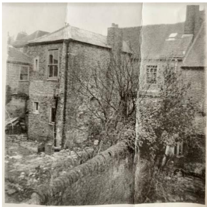
The adjacent photograph shows a historic 2- storey extension to the rear of 7 Queen Street. This extension has since been demolished and a new single storey extension built in its place.
