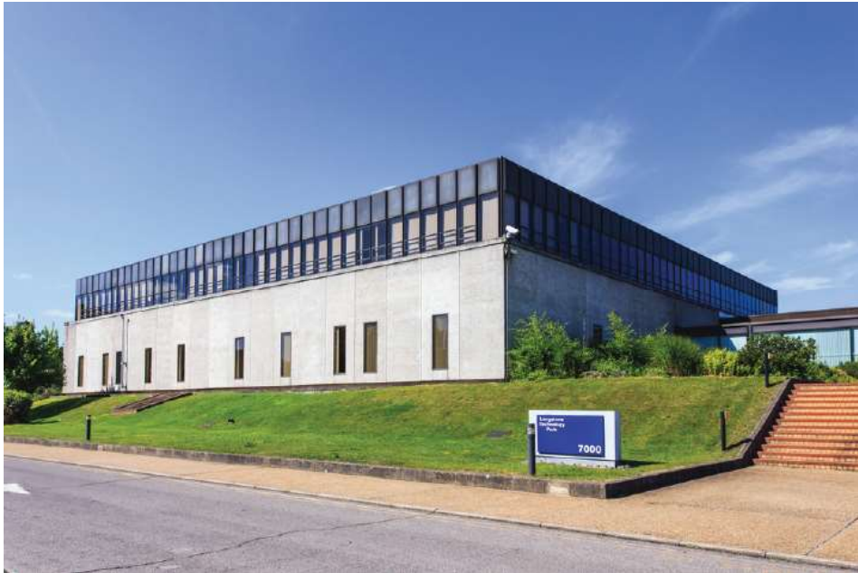
4. View from estate road toward Building 7000
