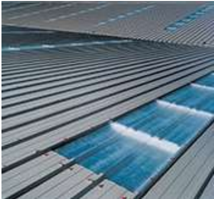
OPTIMISED ROOF LIGHT AREA
