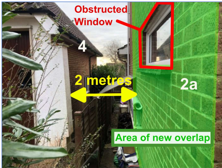
Figure 6. View between property 2a and 4 looking South. Showing current distance of 2 metres between properties, the area in green will be obscured by the proposed property on plot 2 and the window marked in red will be completely obstructed and look onto a solid brick wall to a height of 2 storeys (plus roof)
