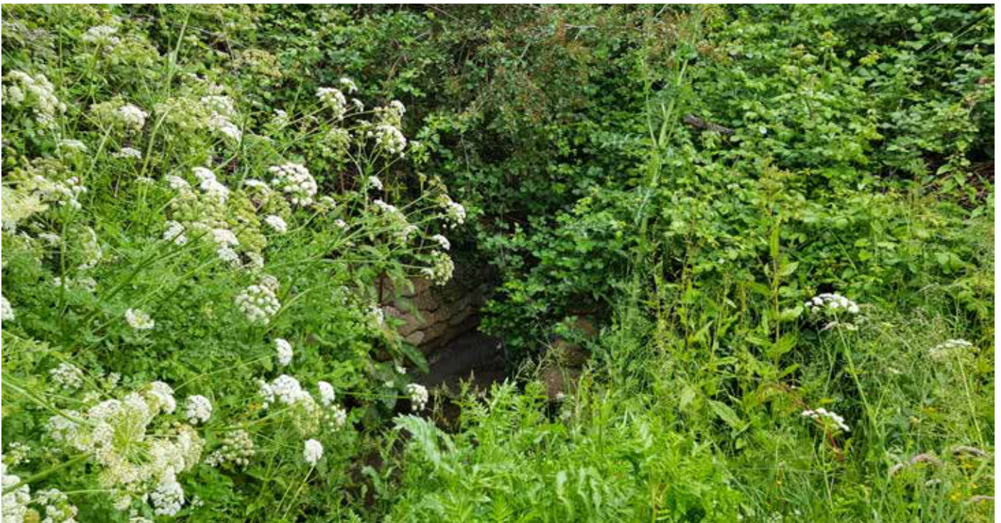
Photograph No. 4 - Southern end of the eastern ditch where it exits the site via an existing culvert.
