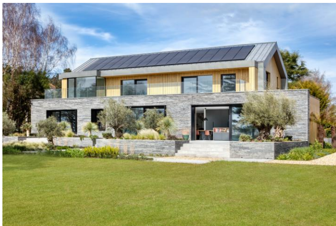
24 Beacon Square – replacement dwelling
