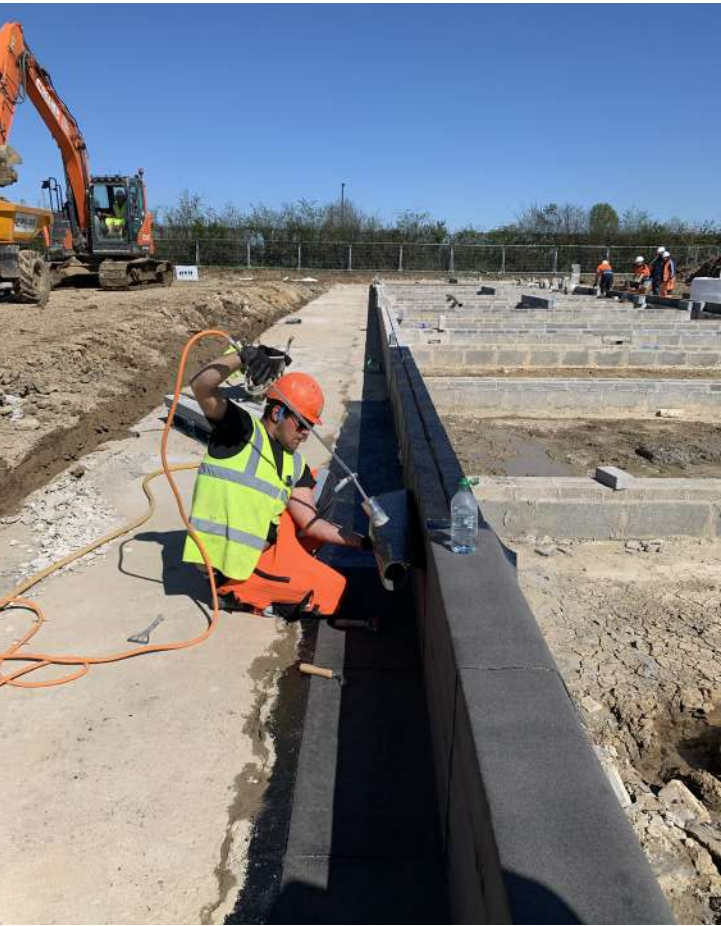
Visqueen torch-on membrane being applied in York
