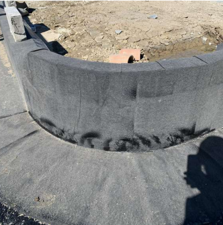
Visqueen torch-on membrane being applied in York
