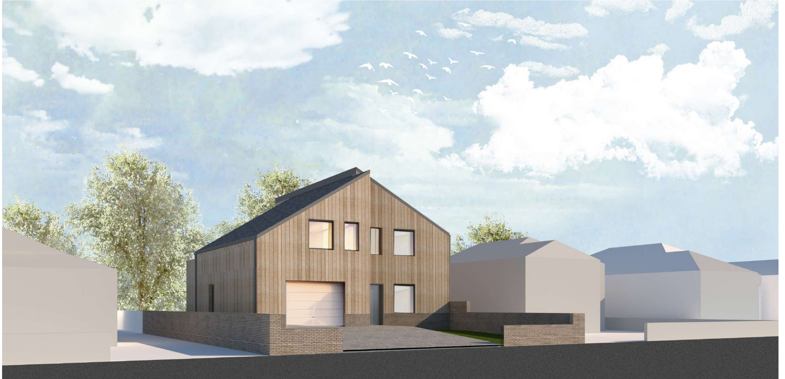
Front view - looking south east
