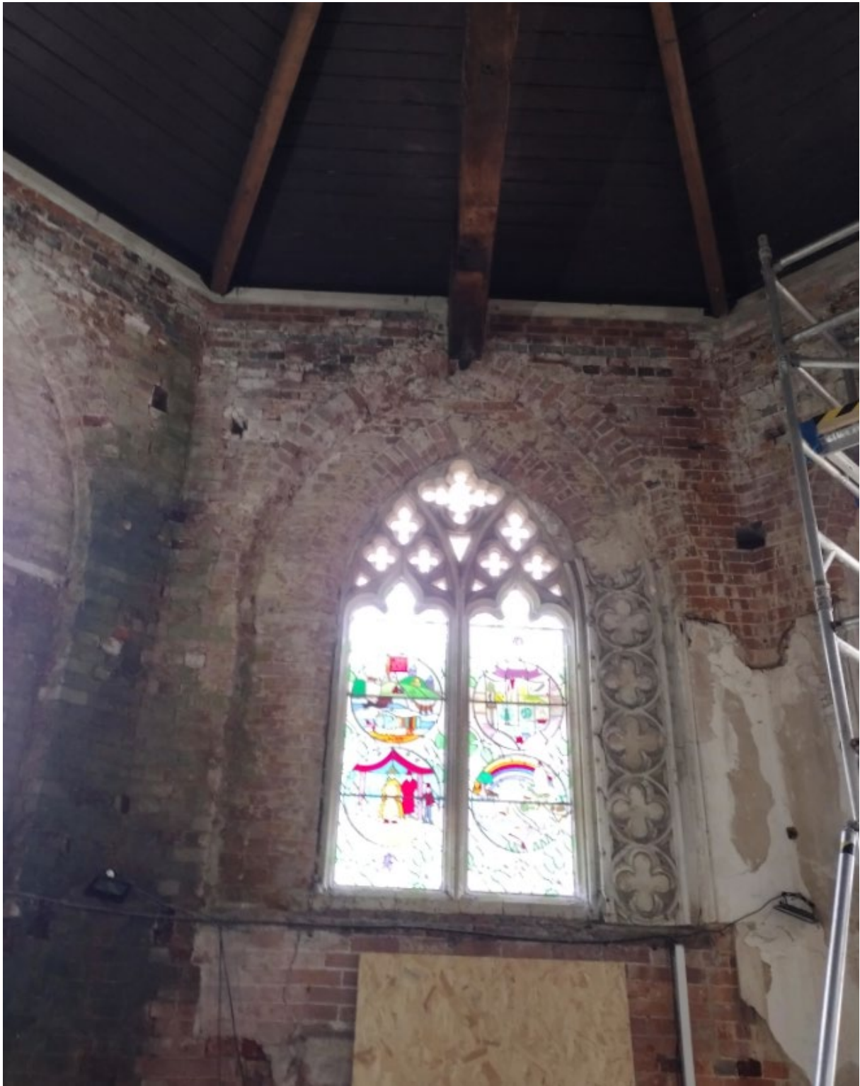
Fig 4: Internal view of Face 5 (North-east).
