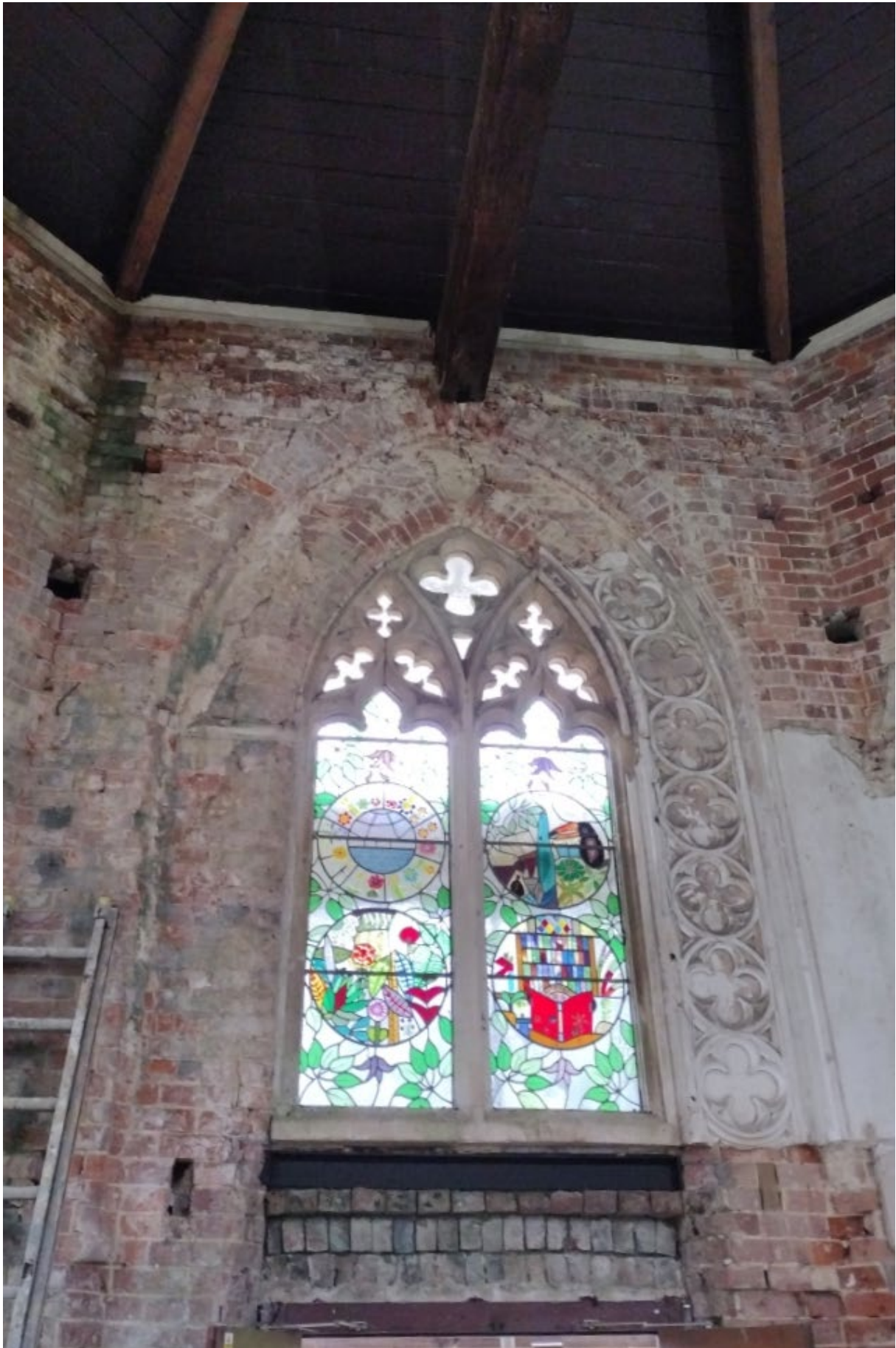
Fig 3: Internal view of Face 1 (South-west).
