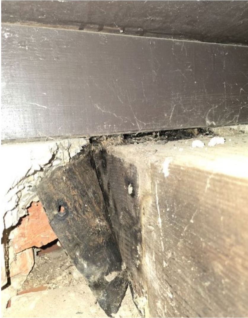
Fig 5: Image showing the end of the main roof beam, and timber wall plate above.
