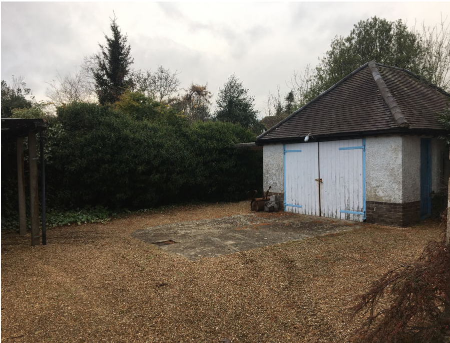
Photograph 02 – B01 is a small garage at the northern end of the site used for storage.
