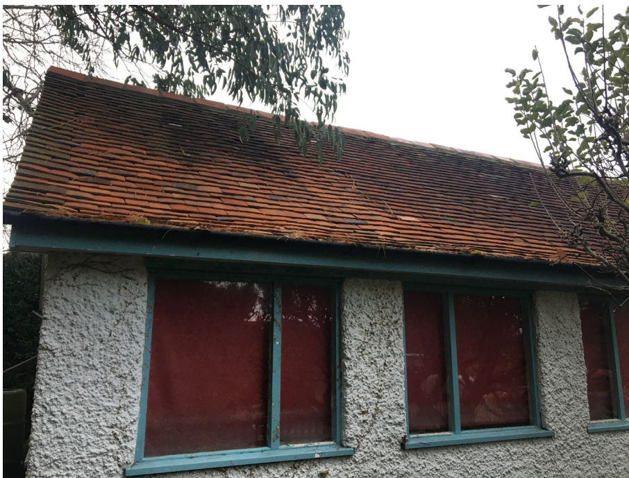
Photograph 04 – The outbuilding (B03) had a vaulted ceiling and was used for storage, viewed here from the west.
