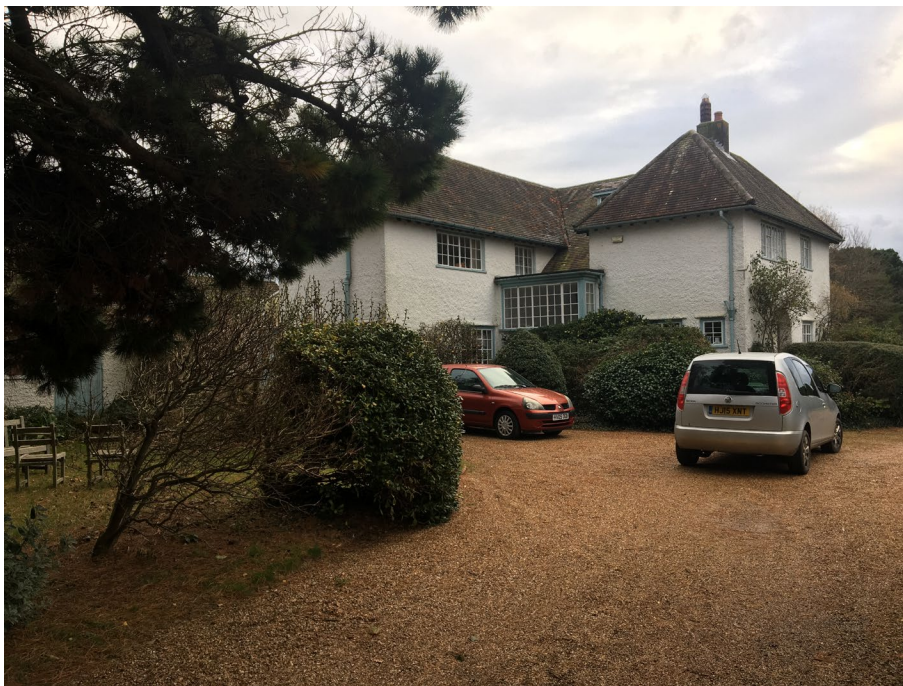
Photograph 03 – The main house located in the north of the site was pebble dashed and had a roof space which had signs of light entering from the outside. Viewed here from the north, the parking area is also obvious.
