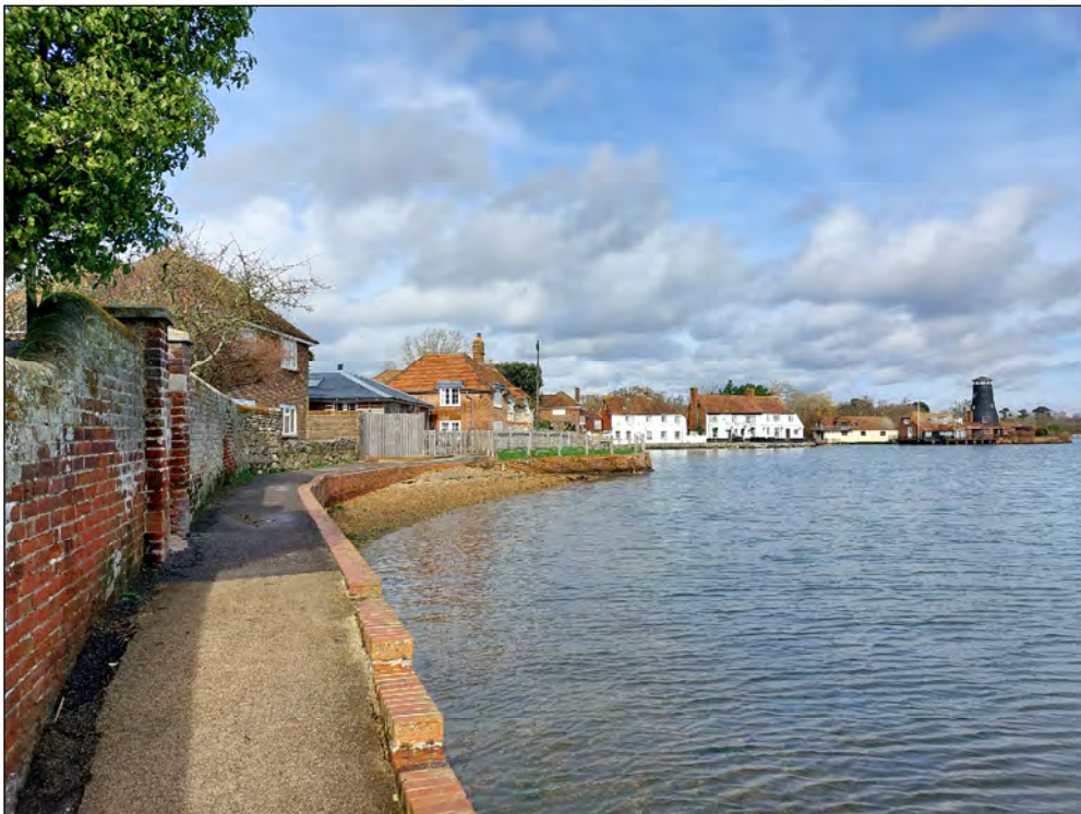
Photo 8) View looking north-east along the southern portion of the Frontage 4 harbour front
