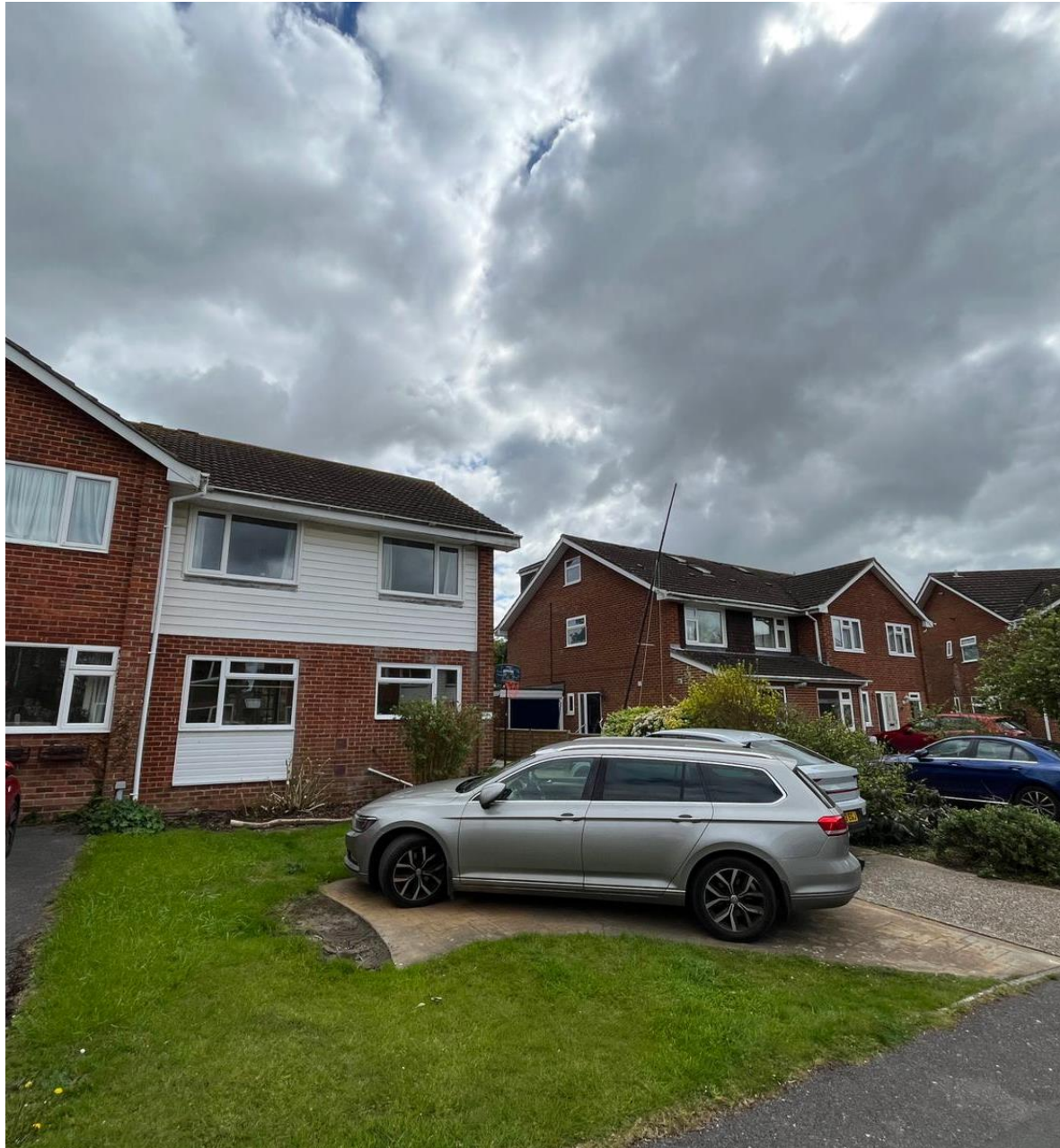
View to front of property from Brook Gardens
