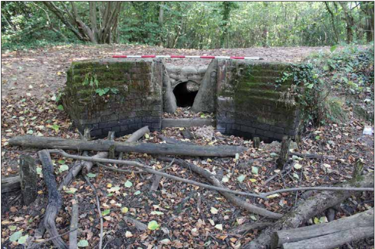
Plate 2: North facing culvert and sluice
