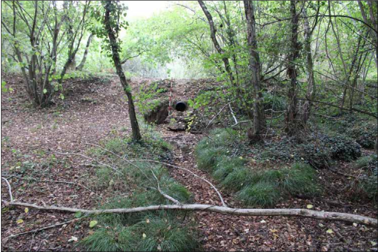
Plate 3: South facing culvert
