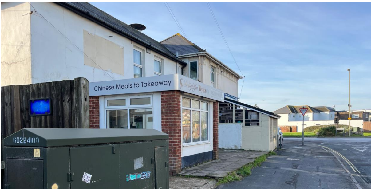
Figure 7 Single Storey Extensions on South Side of Southwood Road Adjacent Application Site
