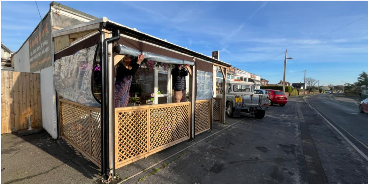
Figure 10 Close Up View of Timber Canopy – Latticed Timber Side Panels; Roll Down Plastic Windows
