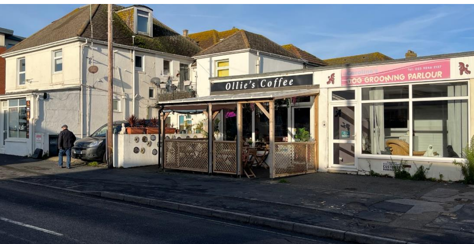
Figure 1 The Front (South) Elevation of Ollie's Coffee
