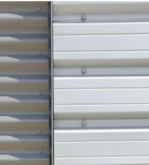
Cladding type 03 & 01 with seperating fin detail
