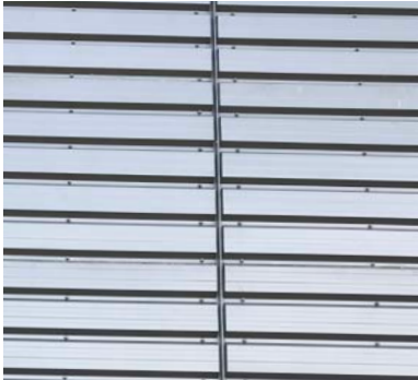
Main body cladding: Trapezoidal profile, laid hori- zontally, Colour: Sirius
