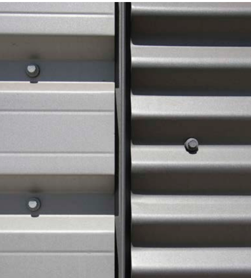
Cladding type 02 & 03 with separating fin detail
