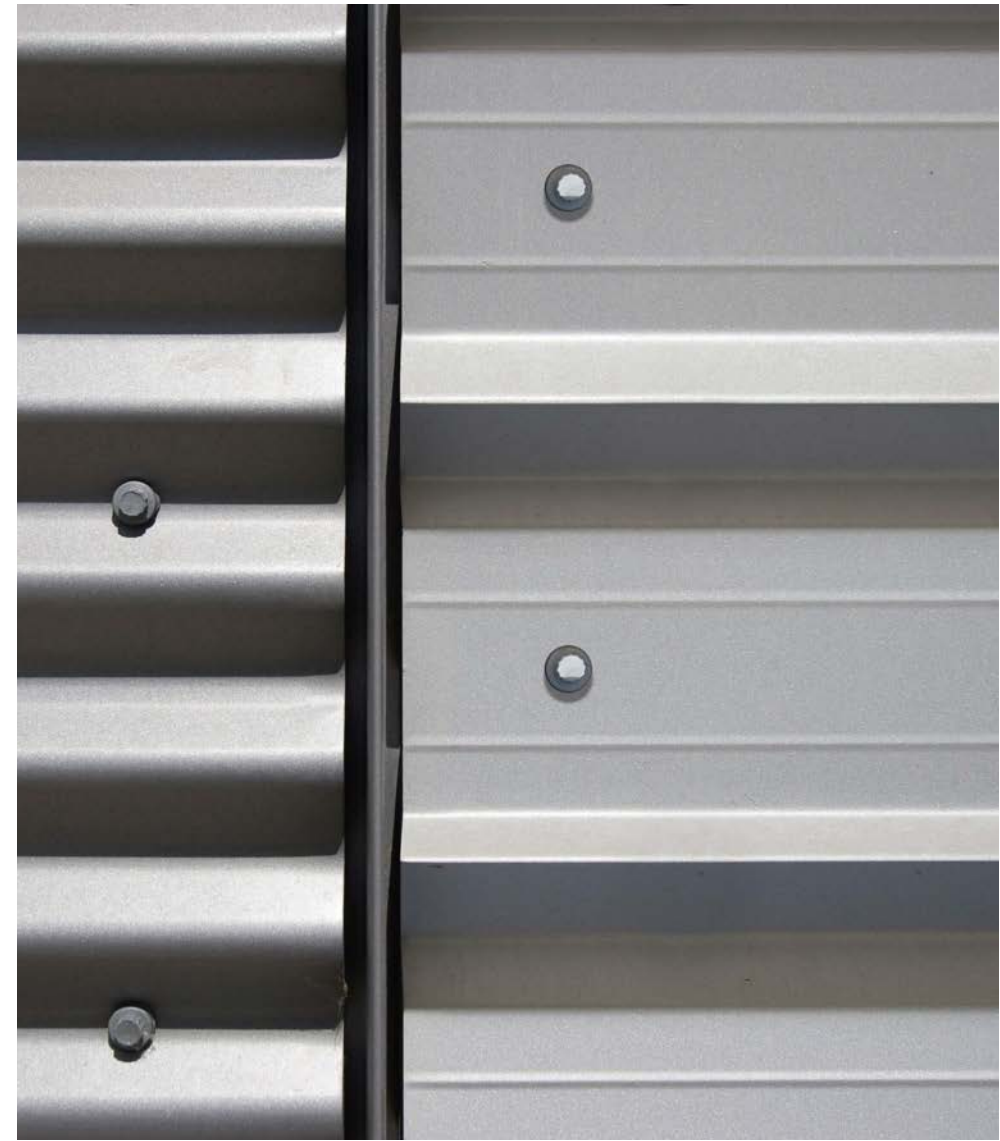
Cladding type 03 & 04 with seperating fin detail
