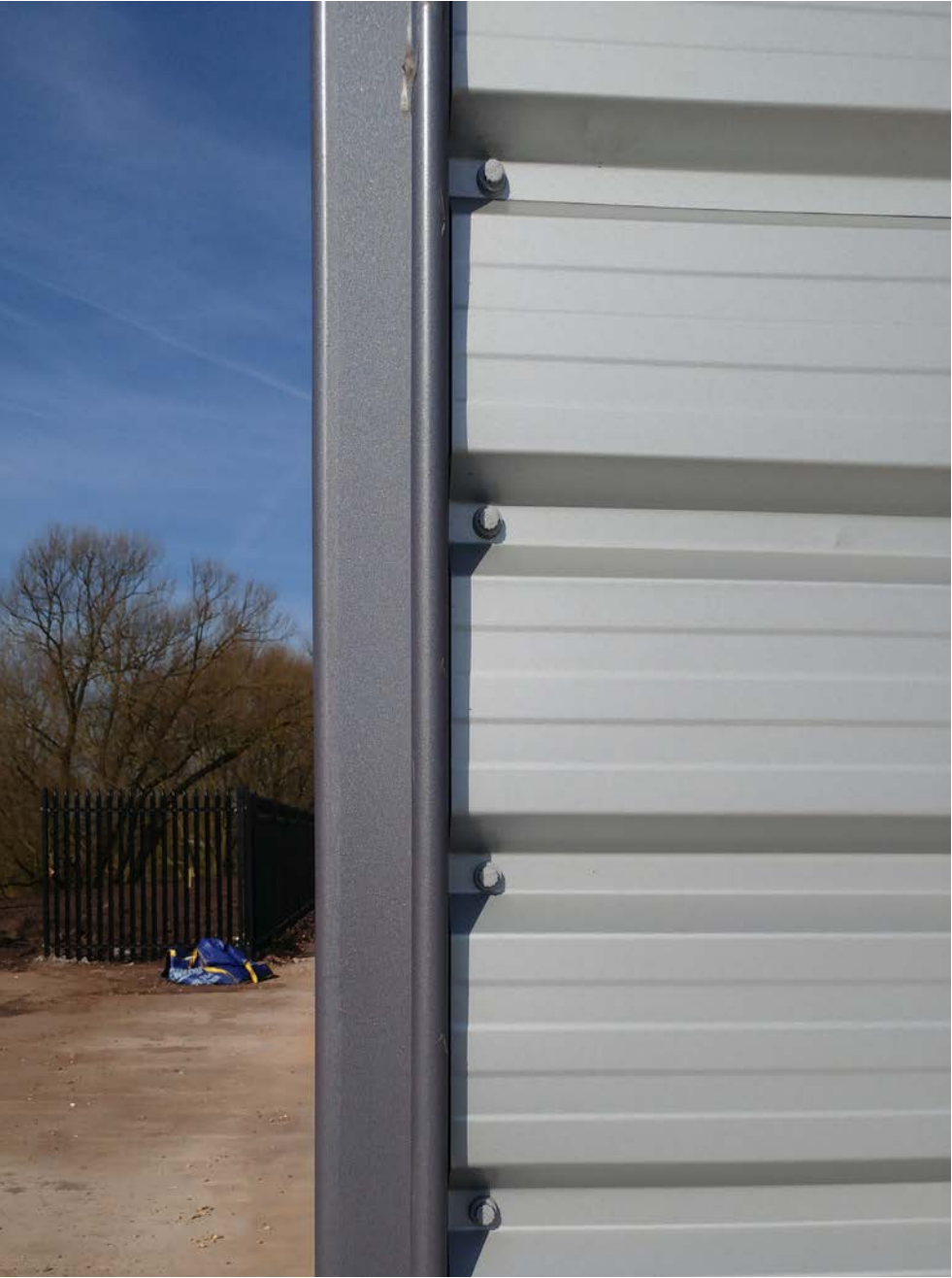
Cladding type 02 & corner fin detail - Precedent image
