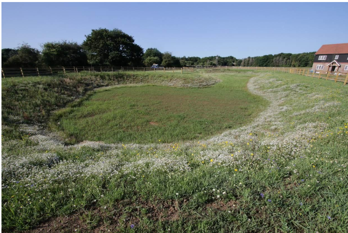
Recently created SUDS feature east of site (July 2023)
