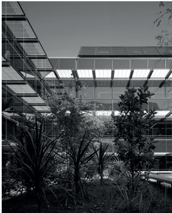
Plate 20: Ground Floor, courtyard, looking south, 1980.
