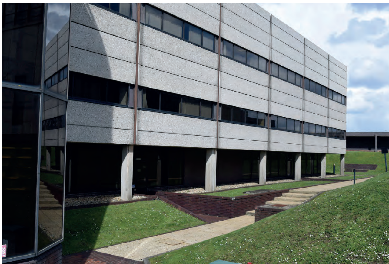
Plate 40: East elevation of Building 6000, looking north- west.
