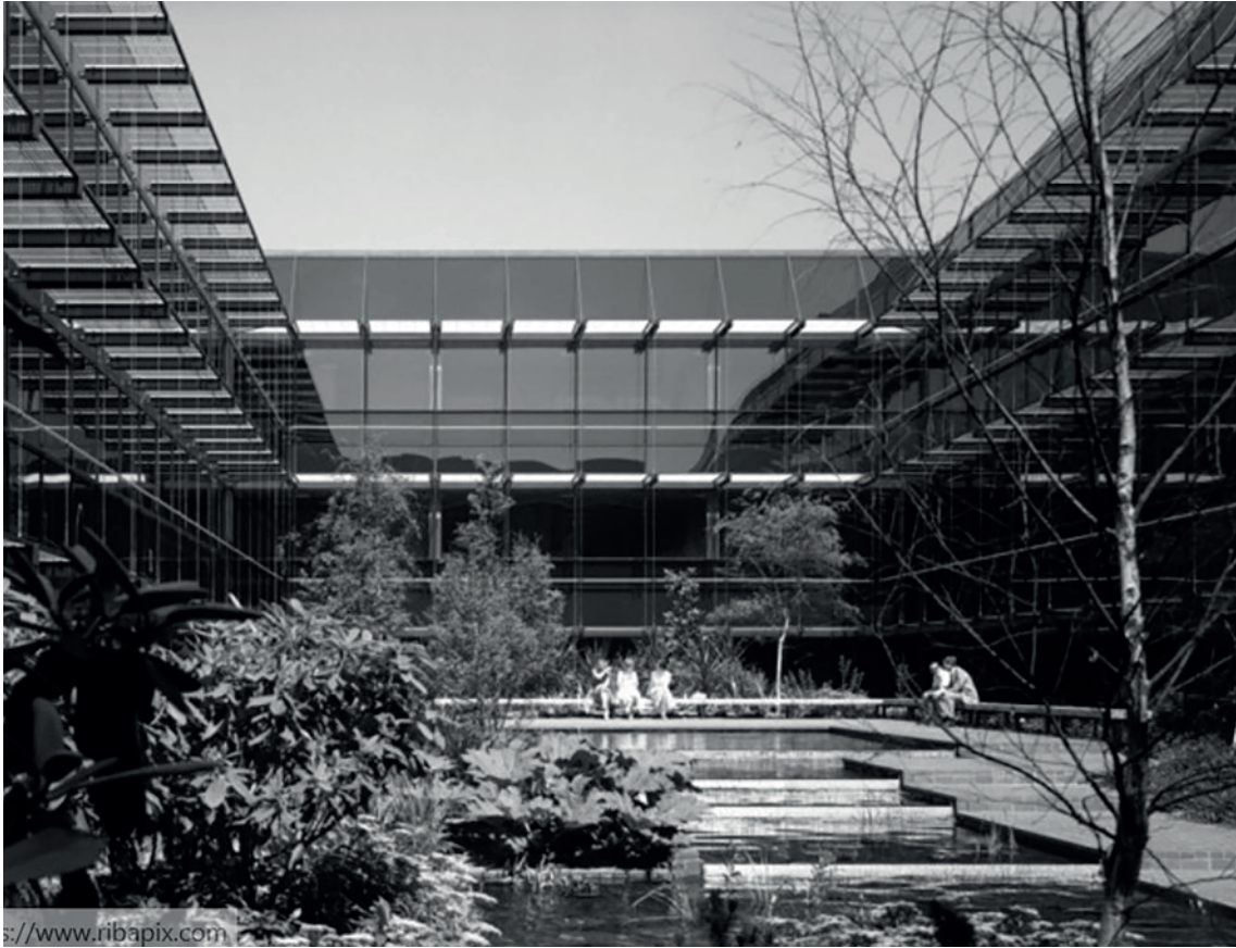
Plate 19: Ground Floor, courtyard, looking north, 1980.
