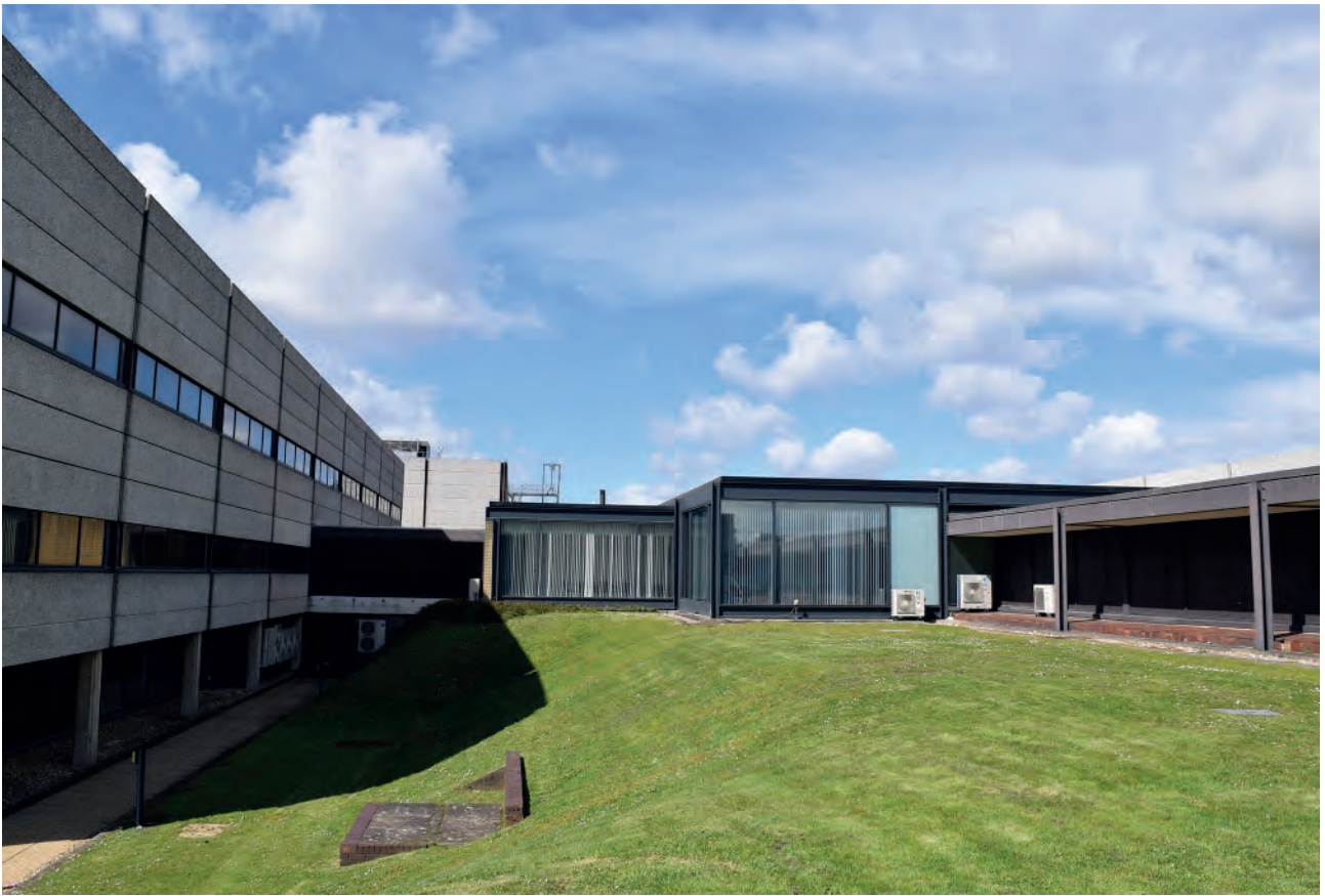
Plate 49: Connection between Buildings 6000 and 4000, looking west.
