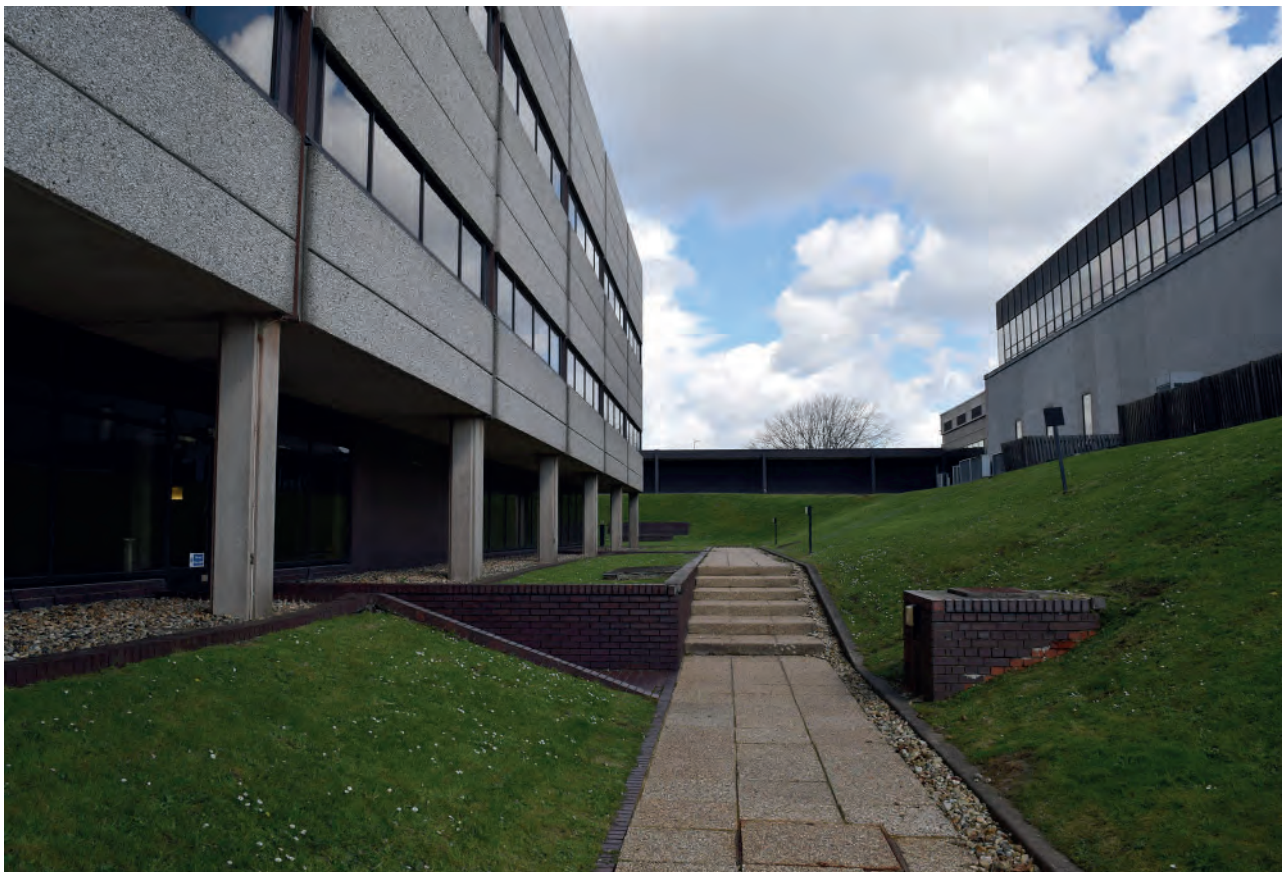
Plate 41: Walkway between buildings 6000 and 7000, looking north.
