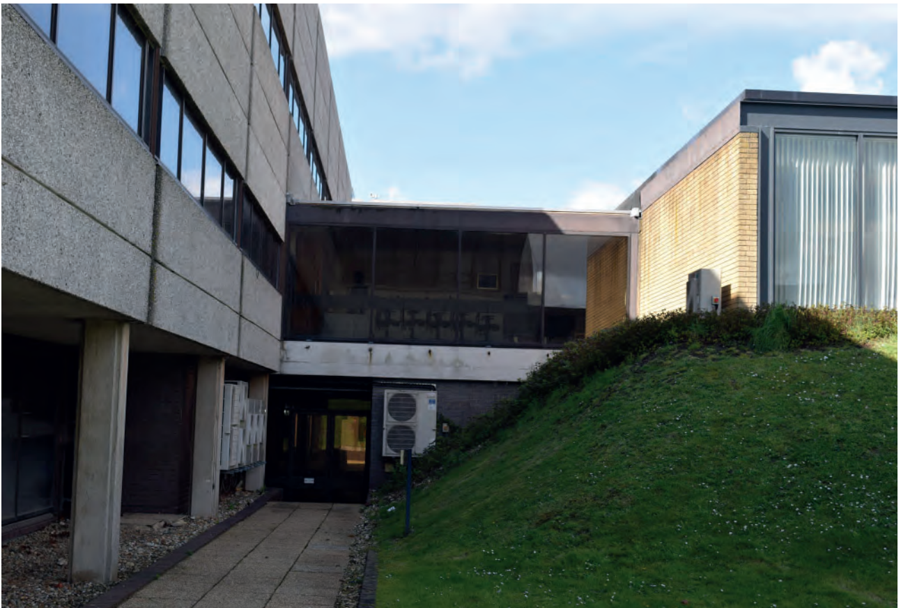
Plate 52: Connection between buildings 6000 and 4000, looking west.
