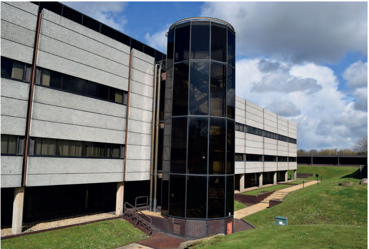
Plate 38: East elevation of Building 6000, looking north- west.
