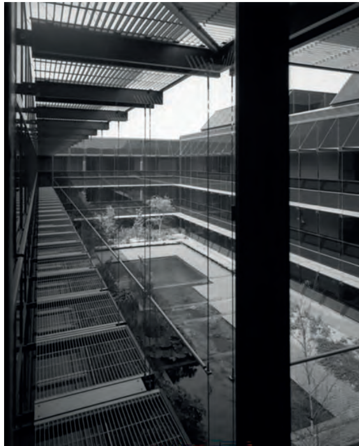
Plate 29: Second Floor, courtyard, looking north- east, 1980.
