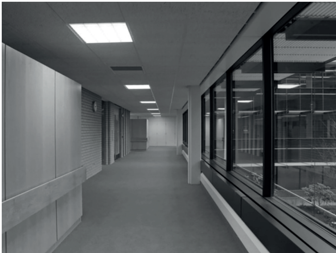
Plate 21: First Floor, south corridor, looking west, 1980.
