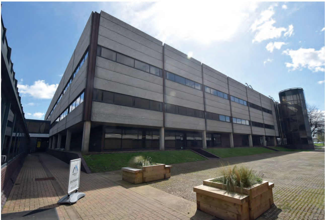
Plate 66: Northwest corner of Building 6000, looking south- east.
