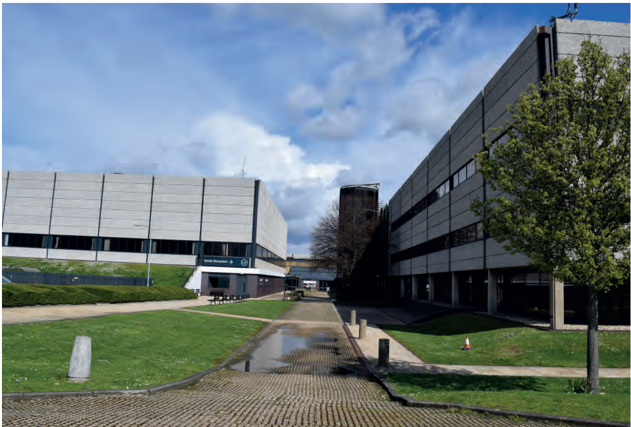
Plate 57: Walkway between Buildings 6000 and 5000, looking north.
