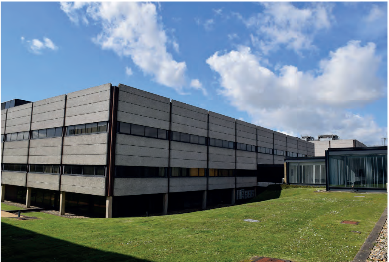
Plate 48: North elevation of Building 6000, looking south- west.
