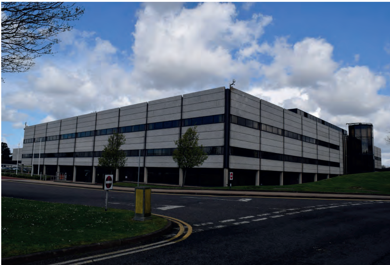
Plate 33: Southeast corner of Building 6000, looking north- west.
