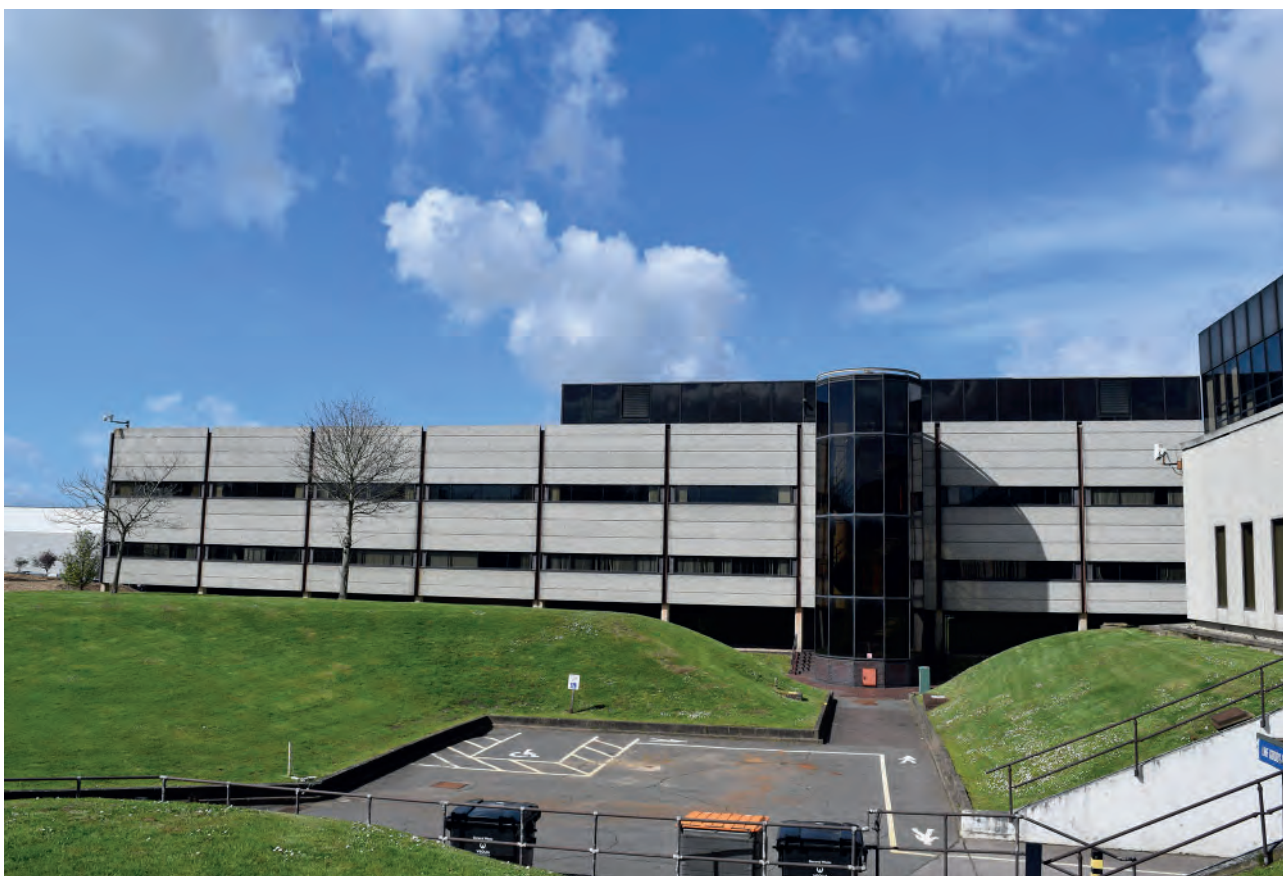
Plate 36: East elevation of Building 6000, looking west.
