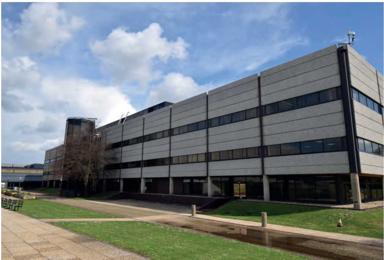
Plate 58: West elevation of Building 6000, looking north- east.
