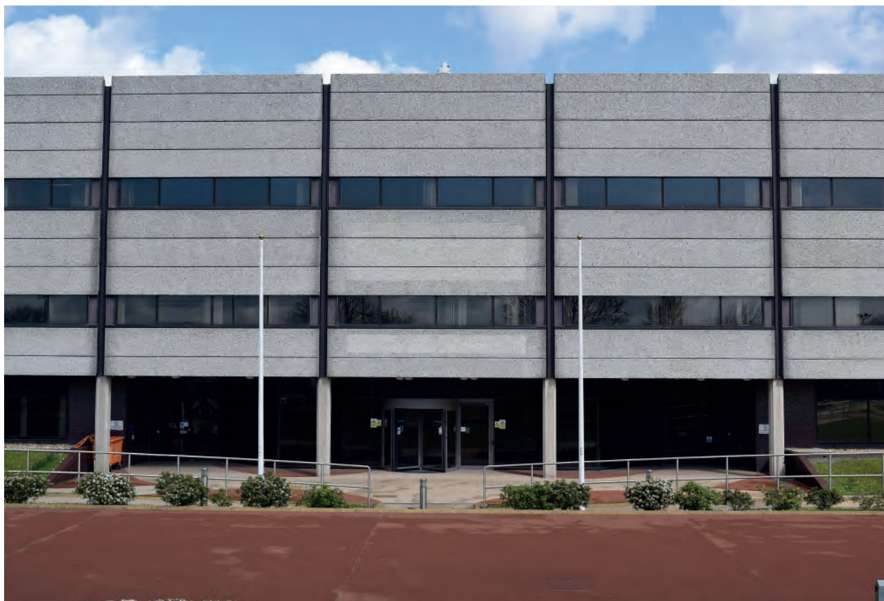
Plate 31: Main entrance to Building 6000, looking north.
