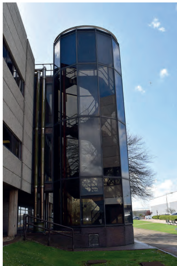
Plate 62: West staircase tower, looking south.
