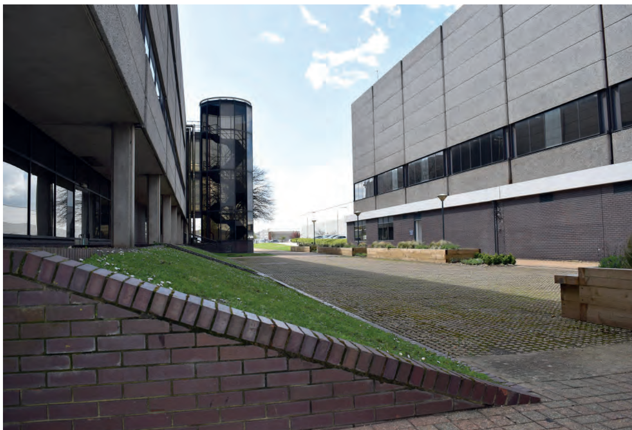
Plate 65: West staircase tower, looking south.
