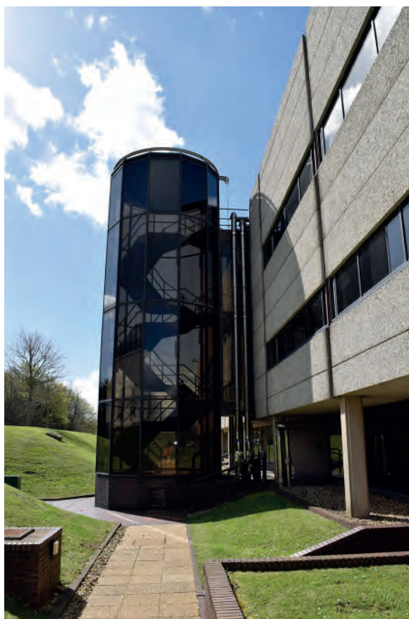
Plate 42: East staircase tower, looking south.
