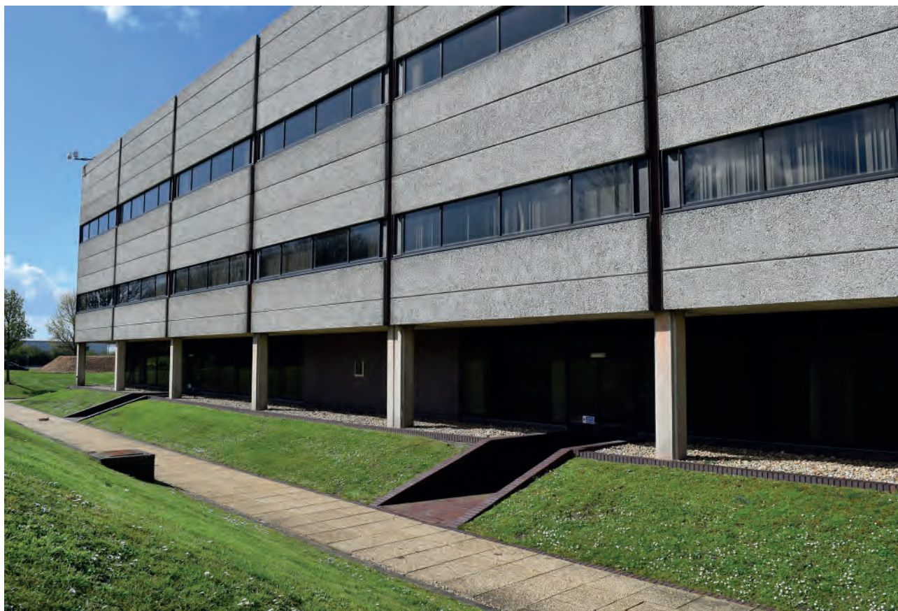
Plate 39: East elevation of Building 6000, looking south- west.
