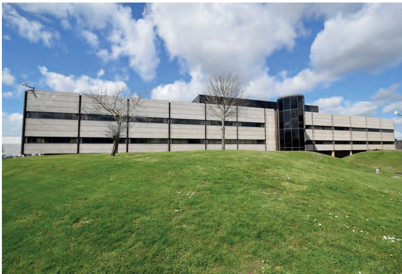
Plate 35: East elevation of Building 6000, looking north- west.
