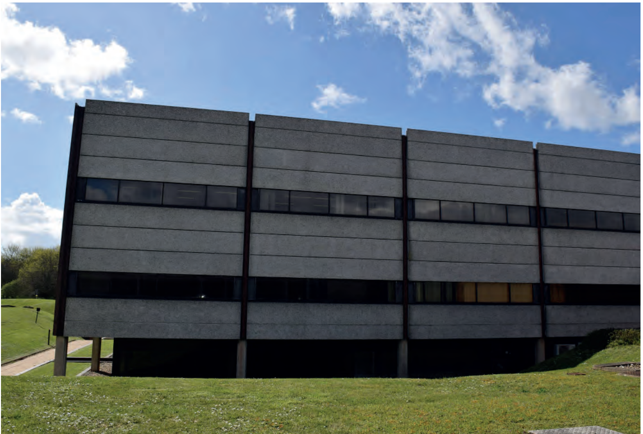
Plate 50: North elevation of Building 6000, looking south.
