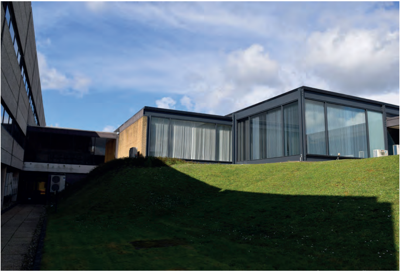
Plate 51: Connection between buildings 6000 and 4000, looking west.
