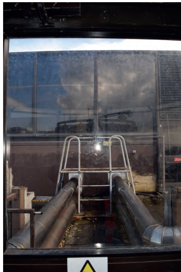
Plate 489: Roof, looking east.
