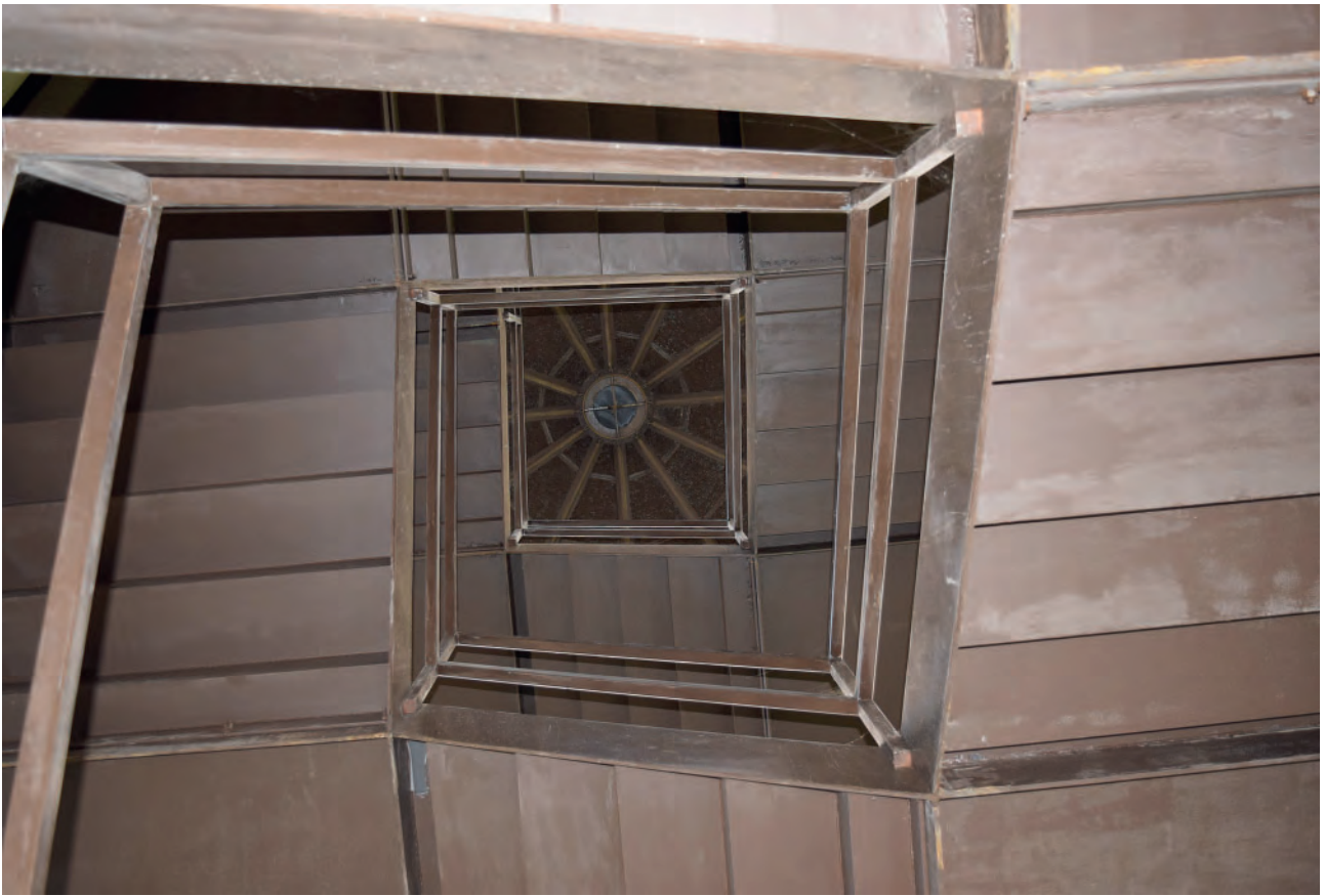
Plate 454: Construction of stairs, ceiling view.
