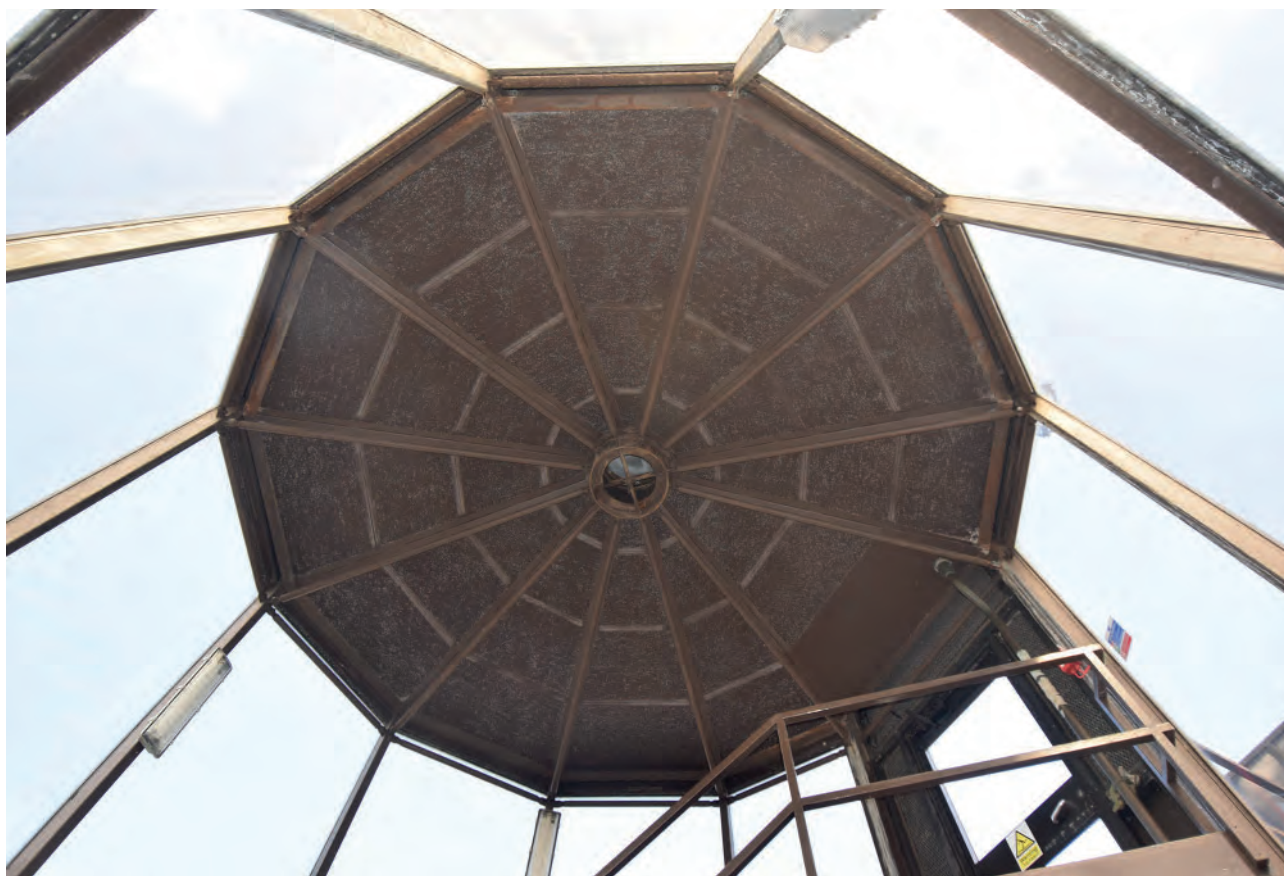
Plate 496: Construction of staircase ceiling.
