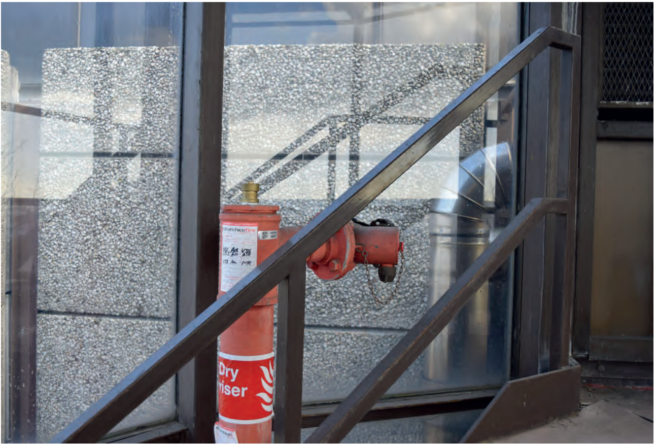
Plate 488: Roof level, hydrant, looking east.
