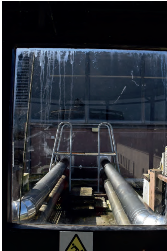
Plate 468: Roof, looking west.
