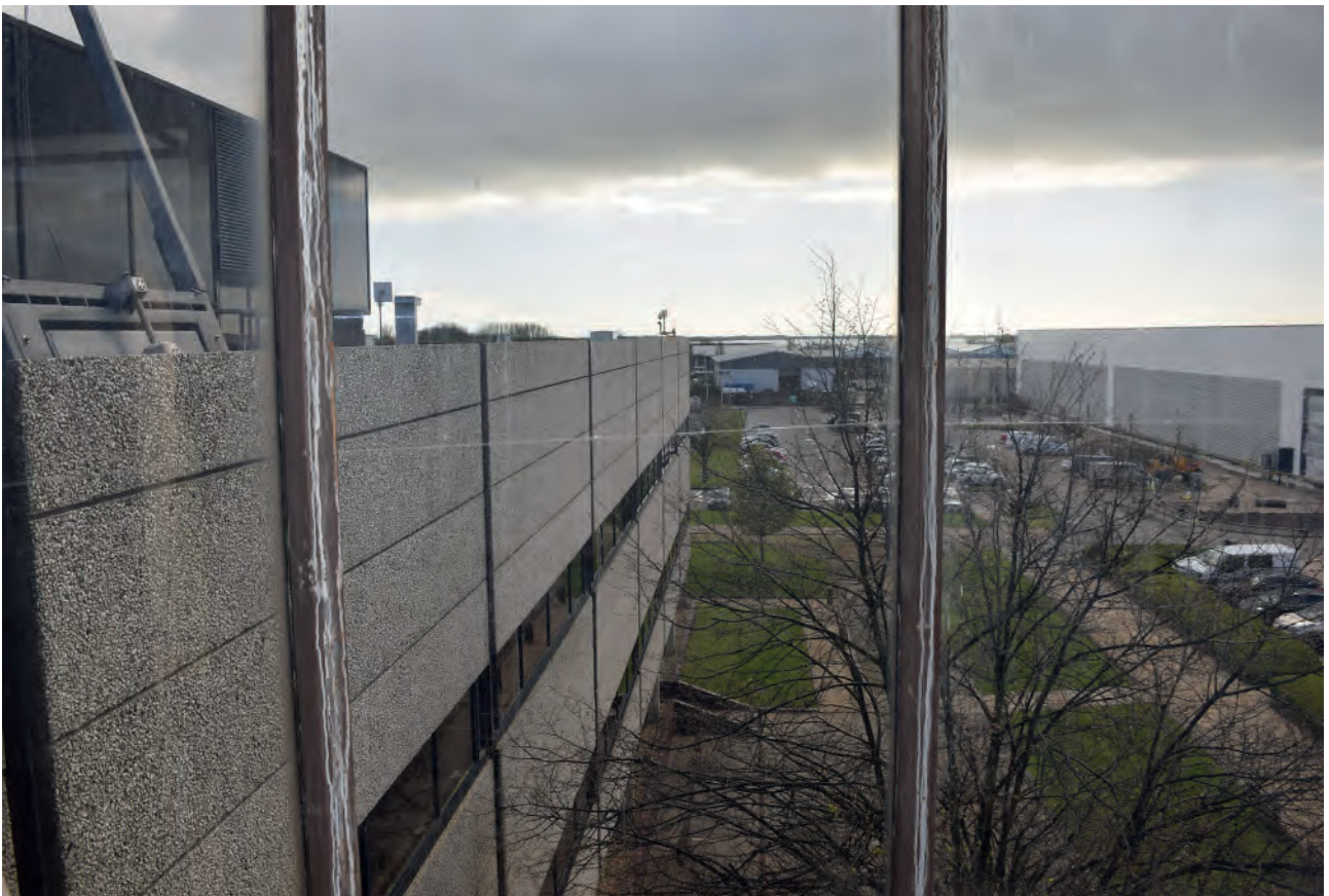
Plate 491: Roof level, looking south.
