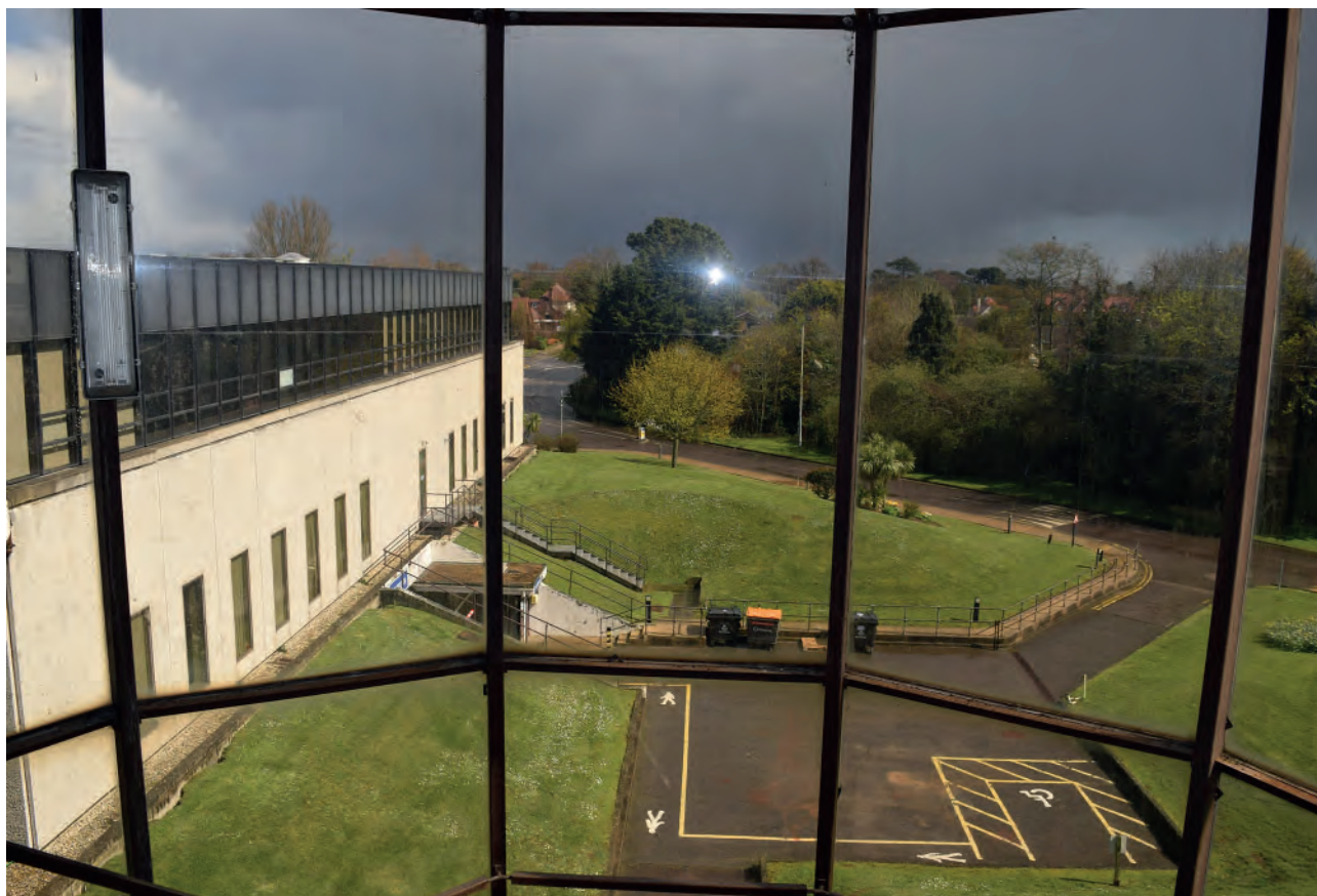
Plate 472: Roof level, looking east.
