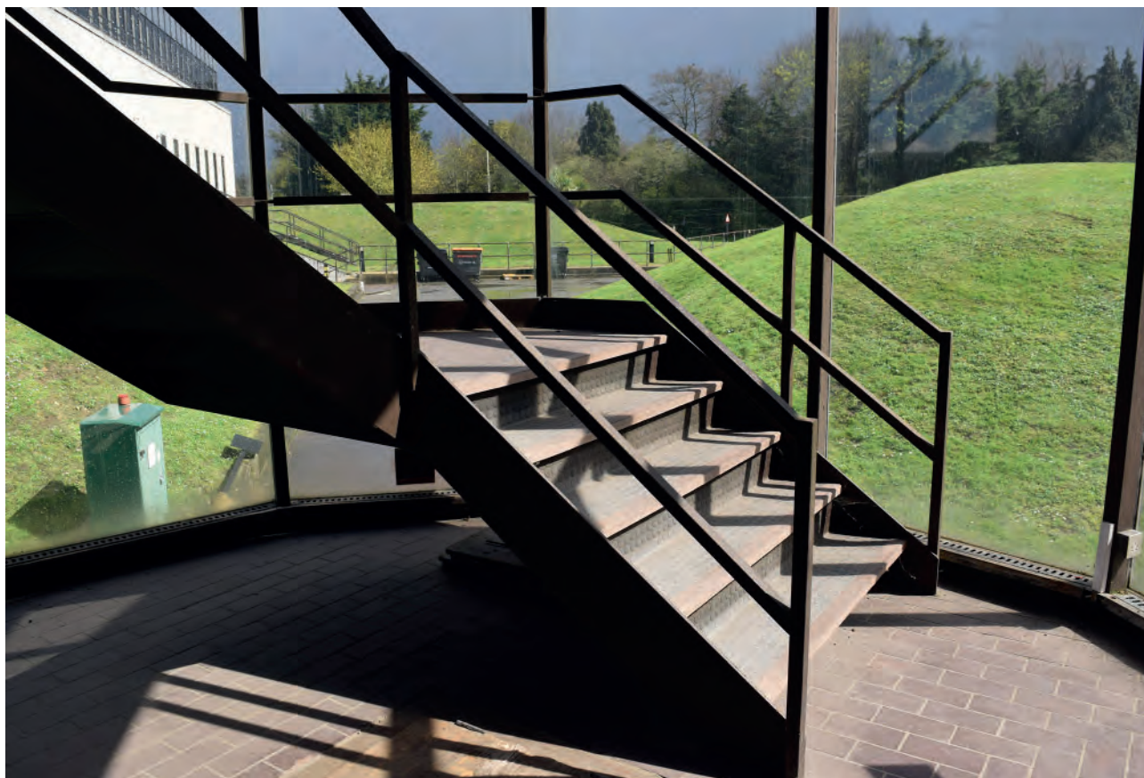
Plate 459: Construction of stairs, looking east.
