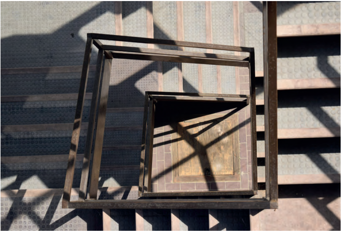
Plate 470: Construction of stairs, ground floor view.
