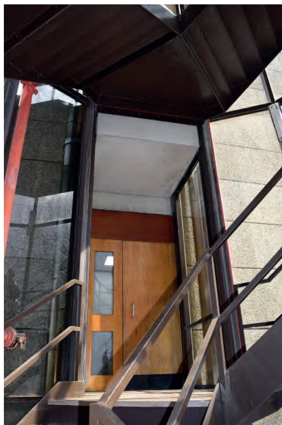
Plate 482: First Floor, emergency door, looking east.
