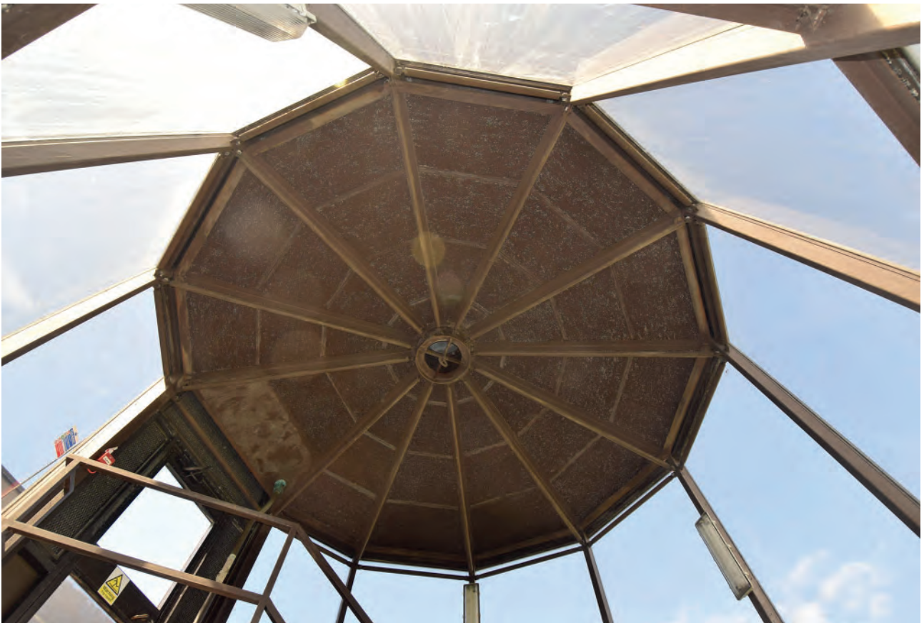
Plate 475: Construction of staircase ceiling.
