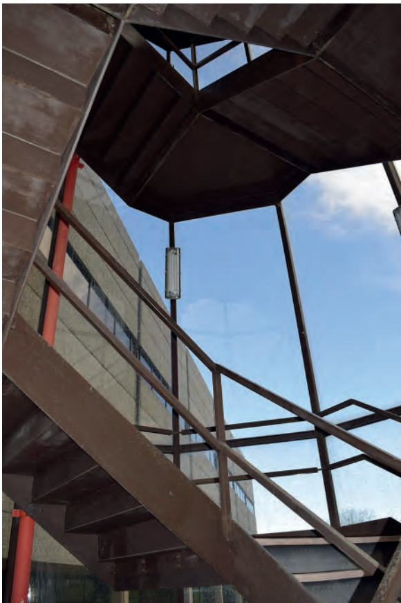
Plate 457: Construction of stairs, looking north.
