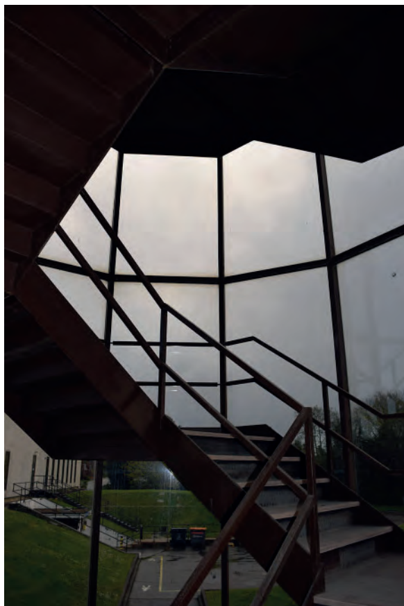
Plate 466 :First Floor, construction of stairs, looking east.
