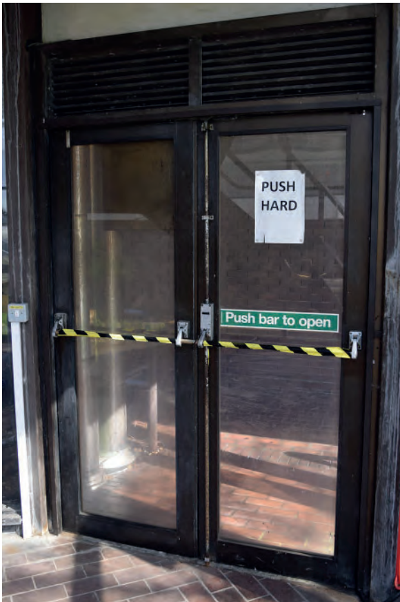
Plate 476: Ground Floor, emergency door, looking east.
