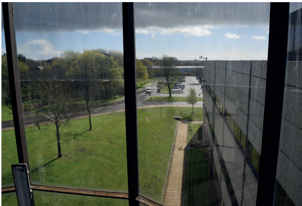
Plate 473: Roof level, looking south.
