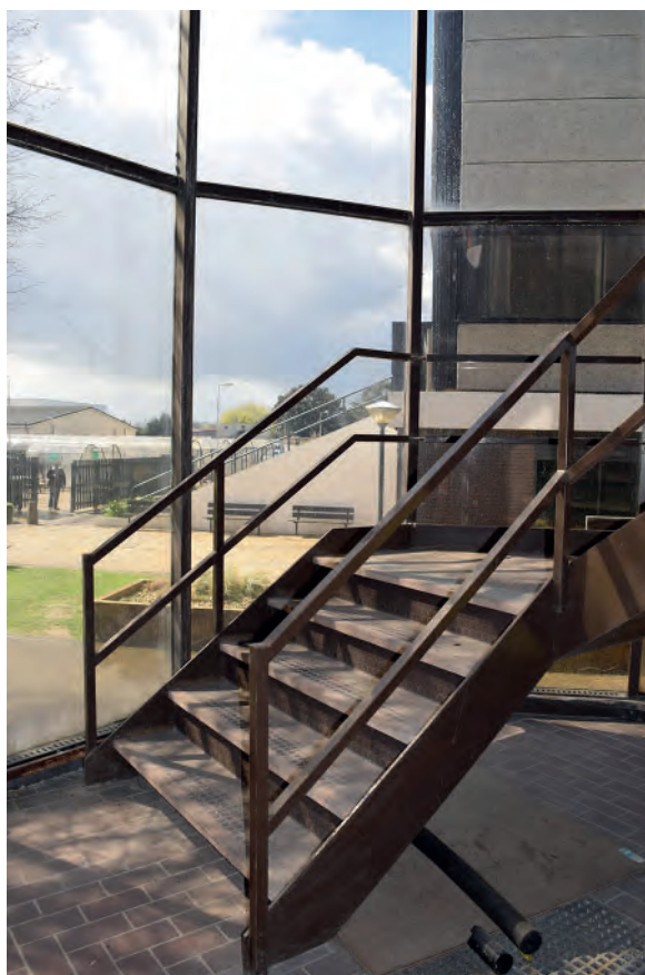
Plate 480: Construction of stairs, looking west.
