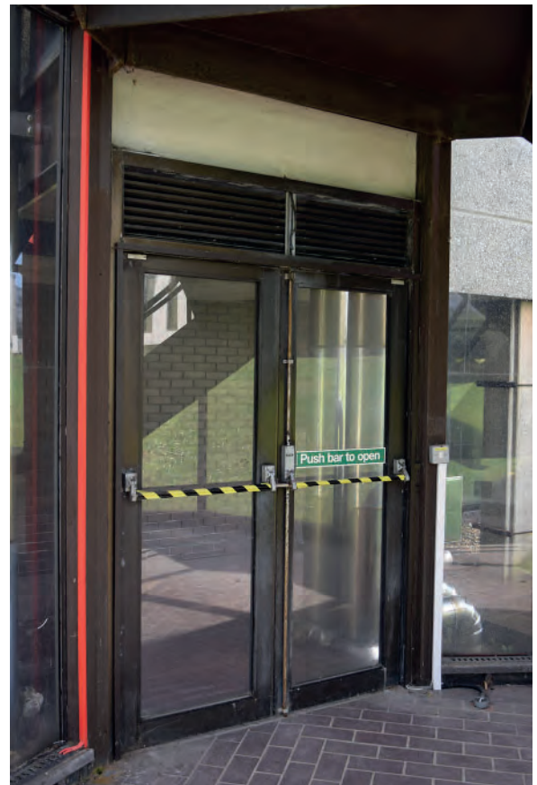
Plate 458: Ground Floor, emergency door, looking north- west.
