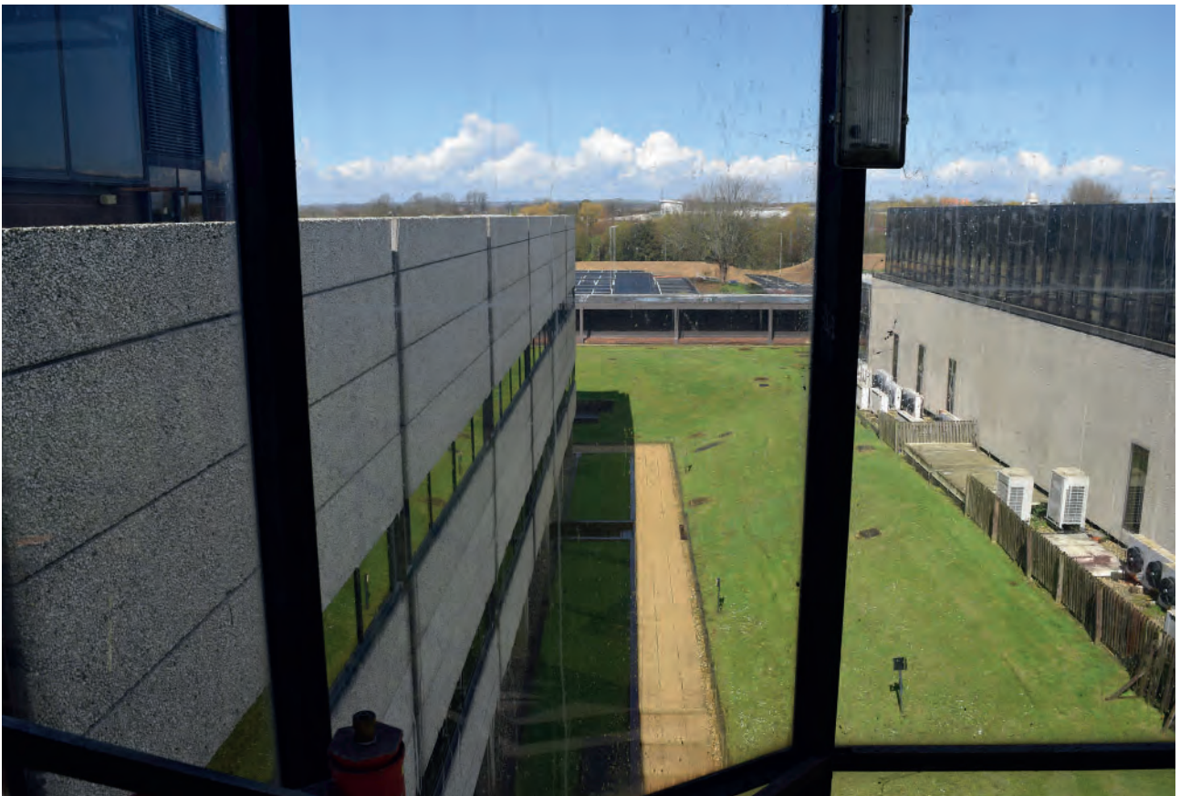
Plate 471: Roof level, looking north.
