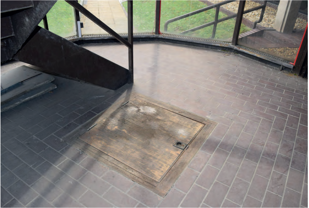
Plate 461: Base of staircase, looking south.
