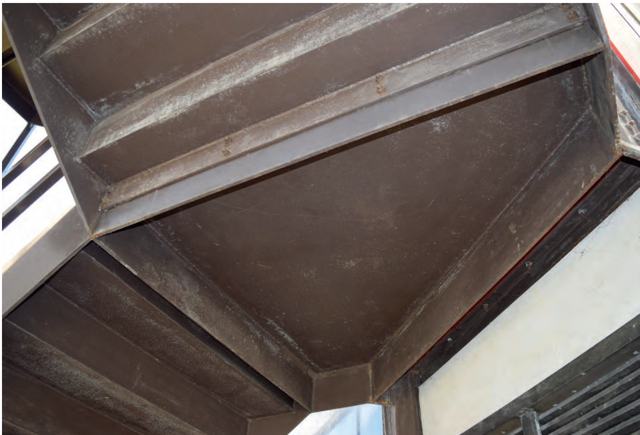
Plate 479: Construction of stairs, landing.
