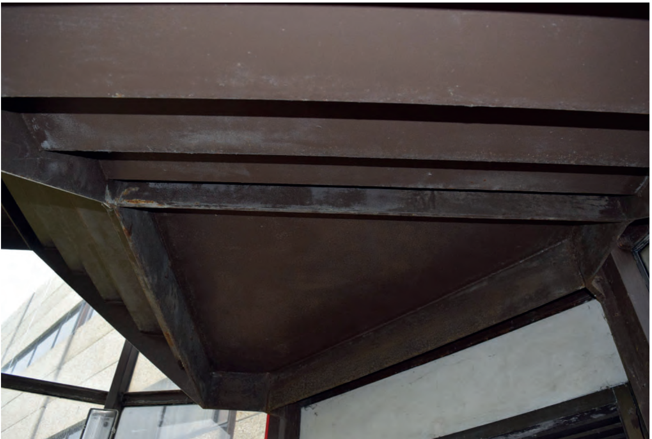
Plate 455: Construction of stairs, landing.
