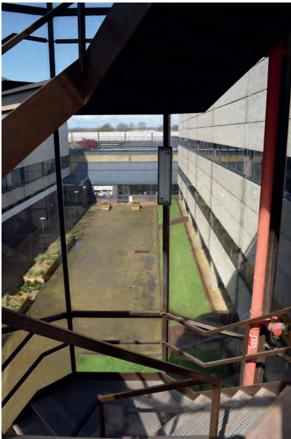
Plate 484: Second Floor, looking north.
