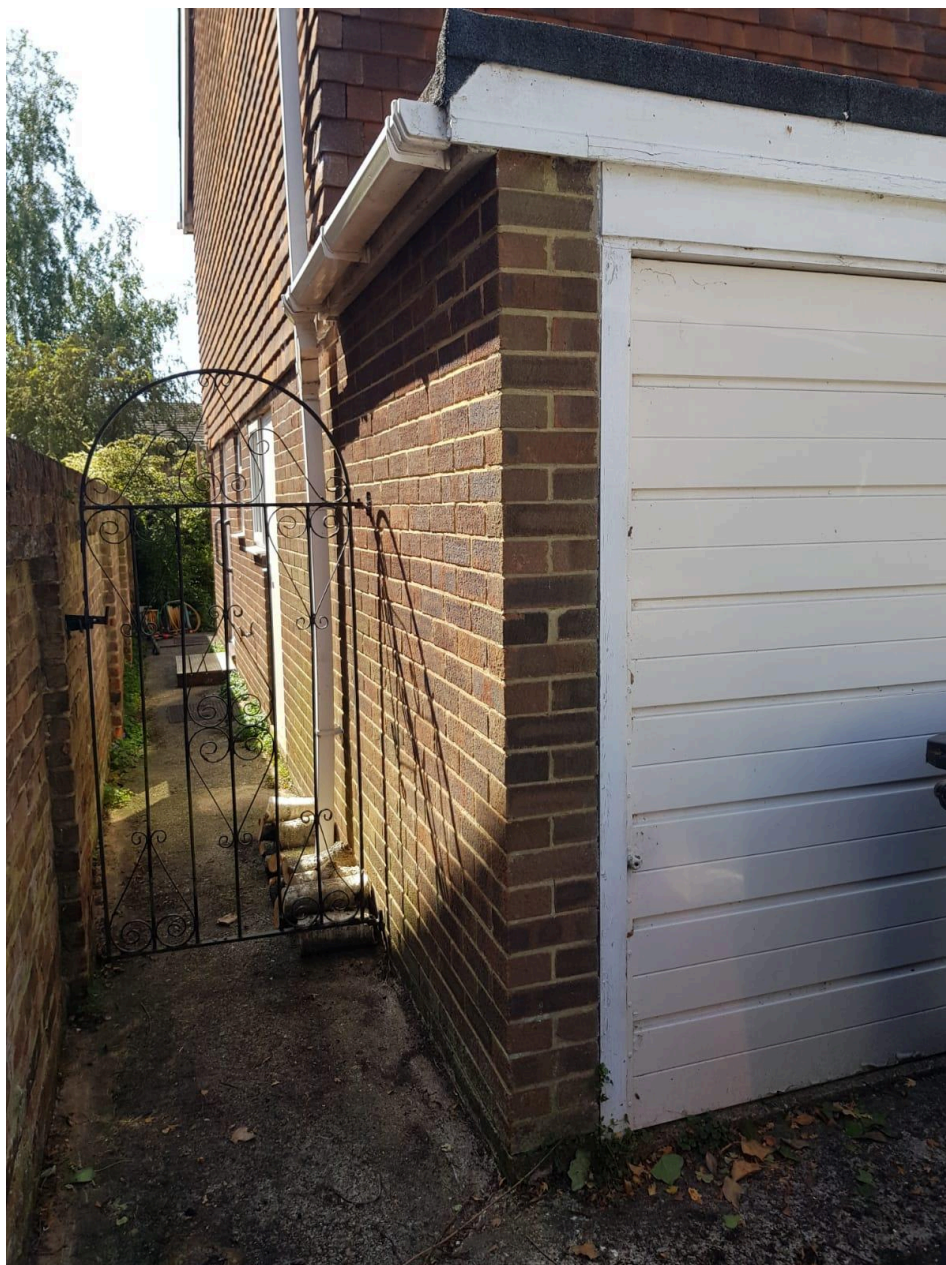
Existing guttering and downpipe
