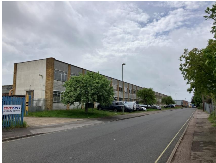
Figure 5. View looking southeast towards T06, T07 & T08
