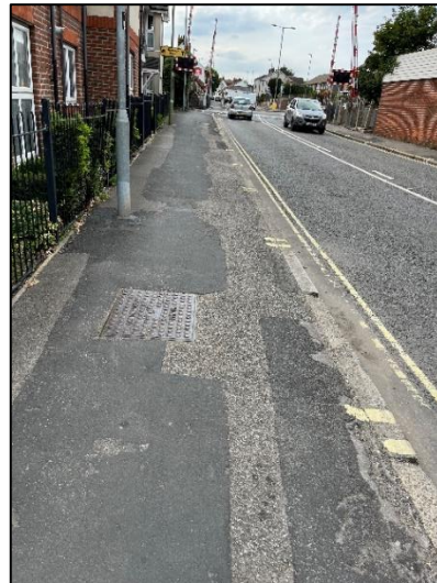
Photograph 3: Footway to Bedhampton Railway Station
