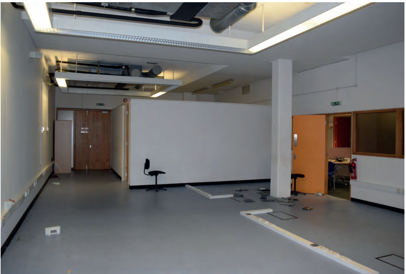
Plate 433: West wing of Building 6000, middle office space, looking south- east.
