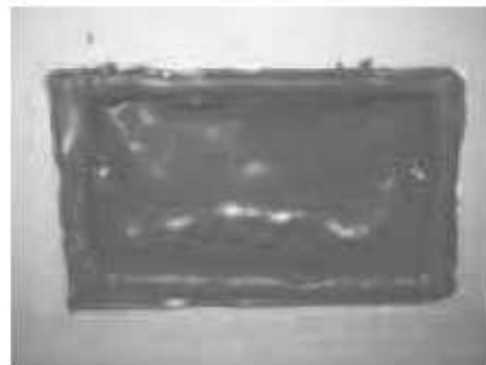
Putty Pad installed inside switch box
