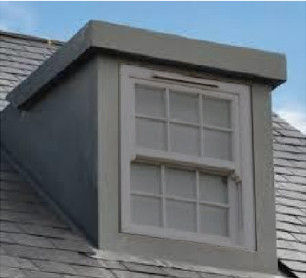
DORMER WINDOW CHEEKS GRP DORMERS IN LEAD GREY COLOUR SIDES AND ROOF
