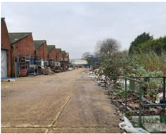
Photograph 4: Hard standing to rear of buildings
