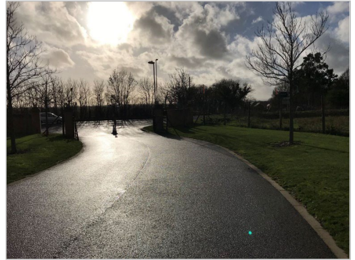
VIEW FACING SOUTH TOWARDS BARTONS ROAD
