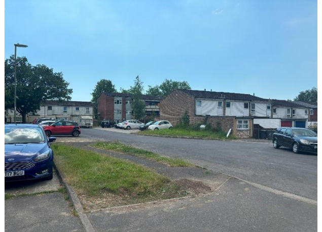
Photograph 2: Existing Conditions along Linnet Close
