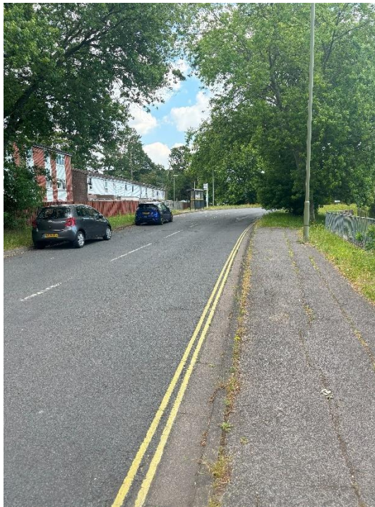
Photograph 3: Existing Parking Restrictions Along Eagle Avenue
