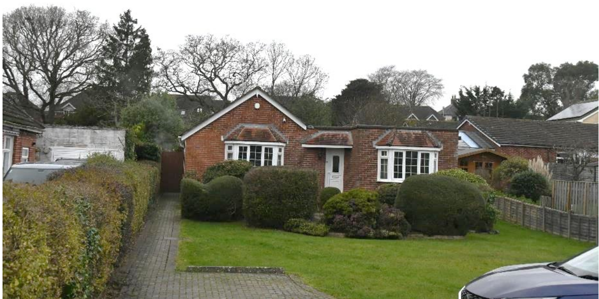
Figure 10: Gable ended and flat roof
