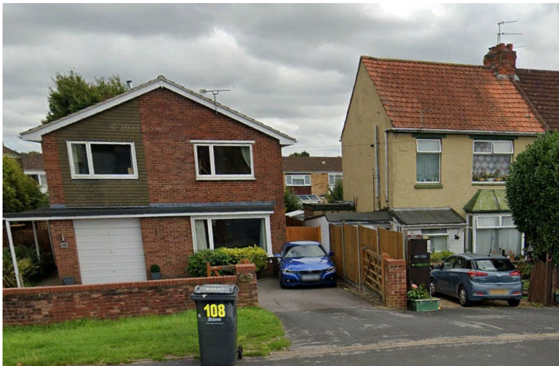
Figure 16: Taller gable end property facing lower gable end property at 90 degrees
