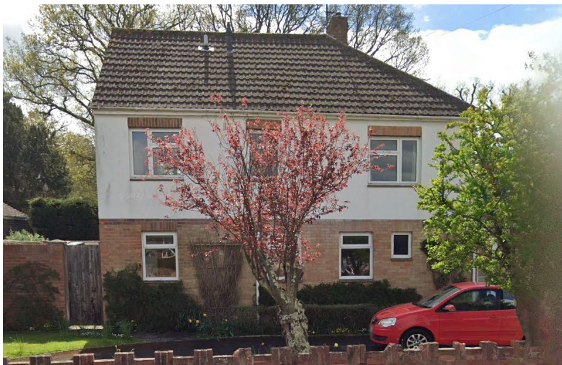
Figure 12: Example of half hip / half gable roof form just outside of the immediate area on Longwood Avenue
