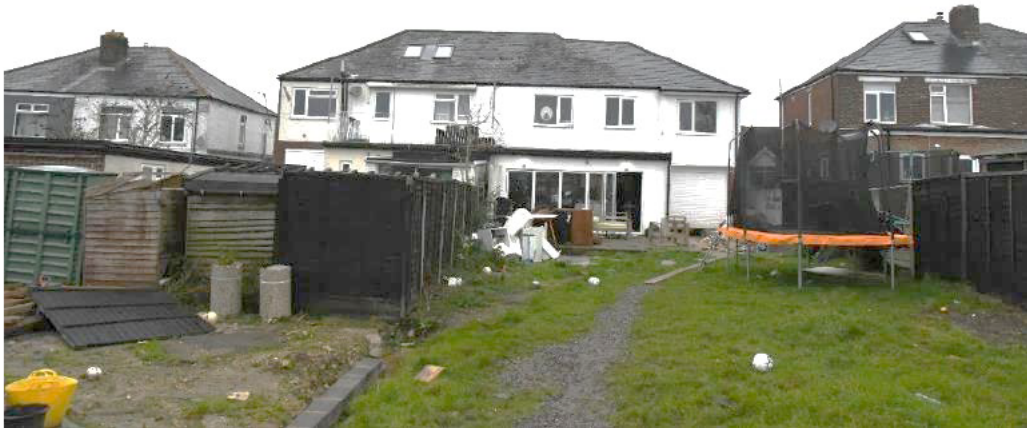
Figure 2: Rear elevation of 28 Gladys Avenue
