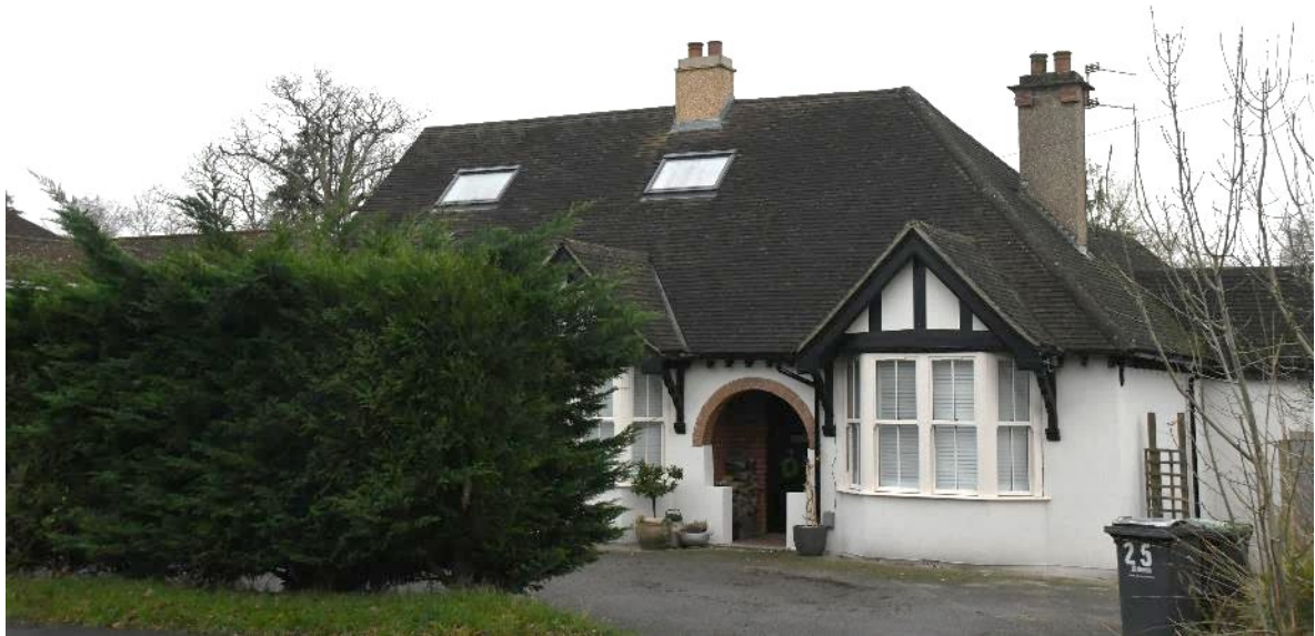
Figure 9: A further example of hipped and gable ended roof
