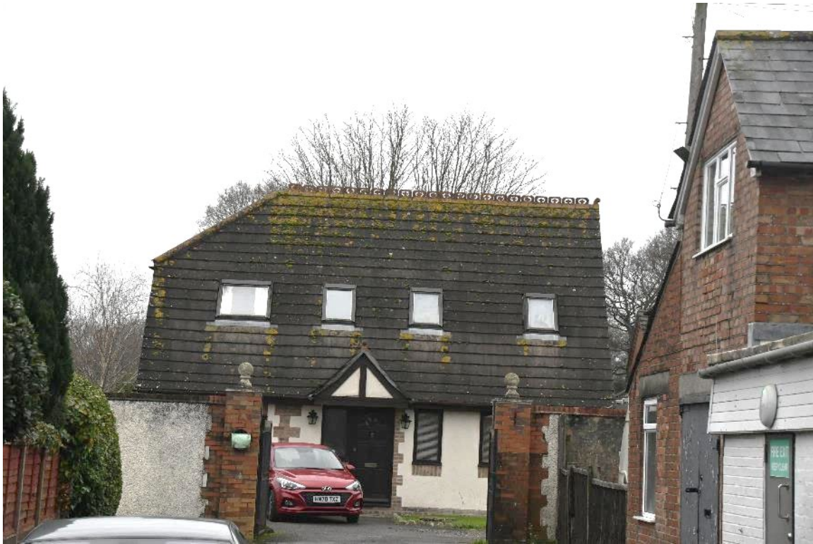
Figure 7: Dwelling with hipped roof on one side and gable end on the other
