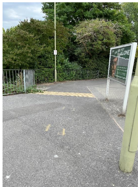
Photograph 63: Shared footway/cycleway heading south from Solent Road
