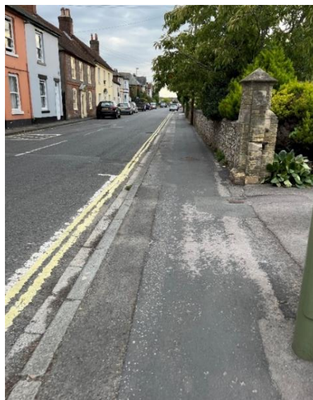
Photograph 24: Northern footway along West Street
