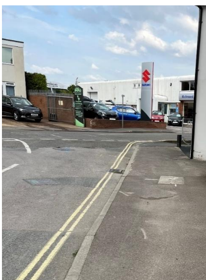
Photograph 10: Vehicular access onto Palk Road and footway along eastern side of the road
