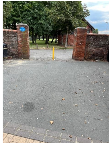
Photograph 51: Access to Havant Park
