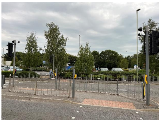
Photograph 66: Staggered crossing across Solent Road
