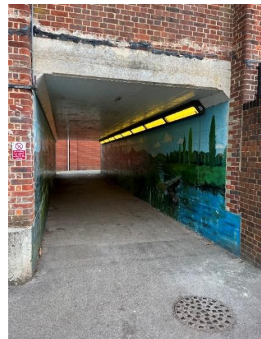
Photograph 55: Underpass from Havant Park
