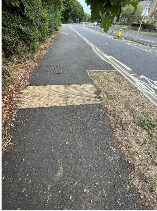
Photograph 38: Footway/cycleway along northern side of New Road
