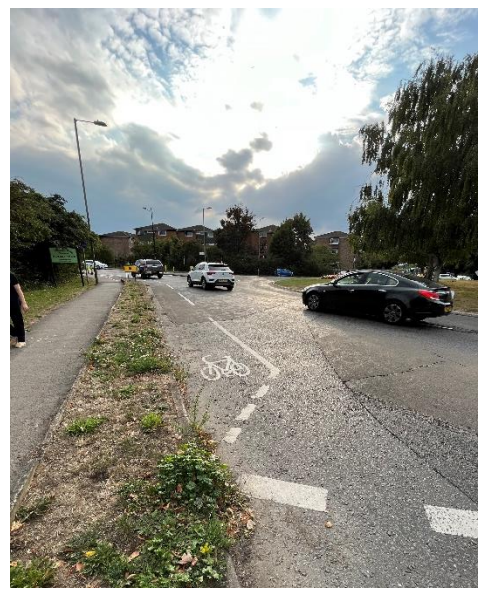
Photograph 43: On-road cycle lane at roundabout junction
