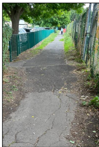
Photograph 20: Conditions of PRoW Footpath 108/507/1
