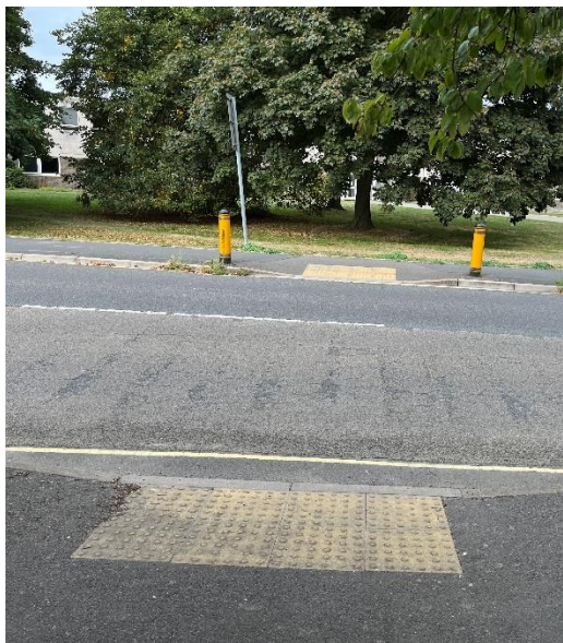
Photograph 42: Elmleigh crossing point
