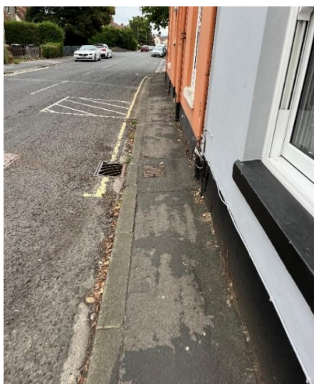
Photograph 23: Narrow southern footway along West Street
