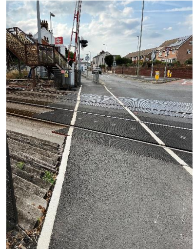
Photograph 14: Pedestrian route along West Street across railway line
