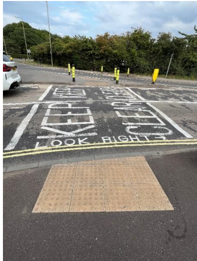
Photograph 40: Park Road North crossing point
