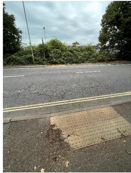
Photograph 69: Crossing point along Solent Road at Solent Road/Brockhampton Road/Marples Way roundabout junction.
