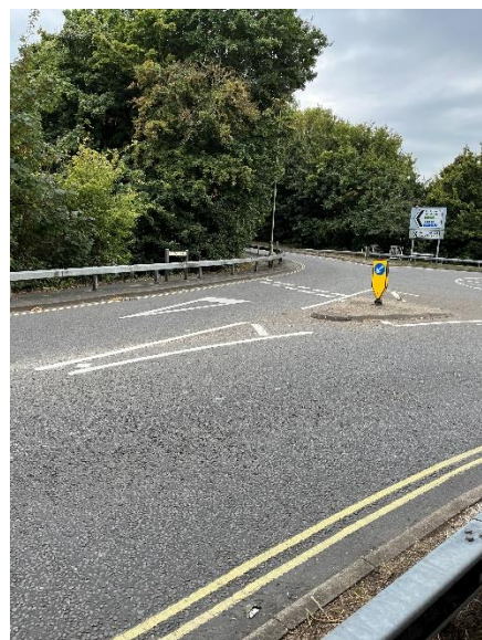
Photograph 71: Vehicle safety barriers at Solent Road/Brockhampton Road/Marples Way roundabout junction
