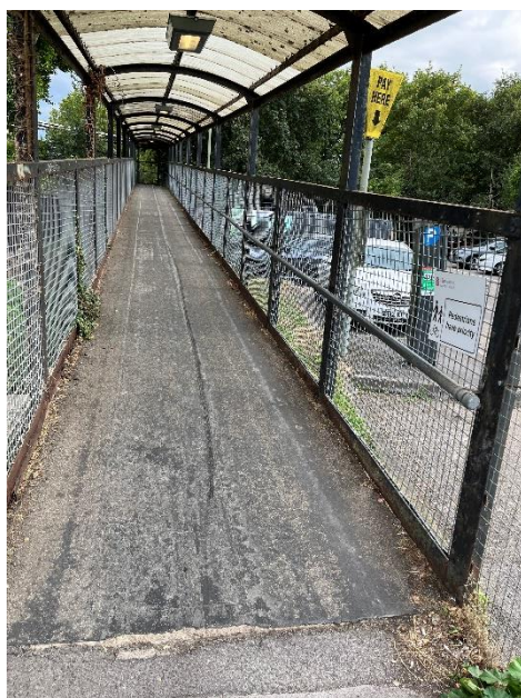
Photograph 44: Footbridge over rail line
