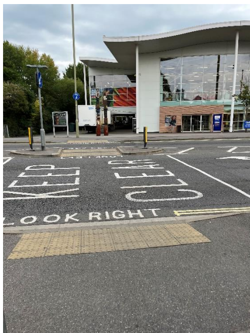
Photograph 62: Uncontrolled crossing point along Solent Road
