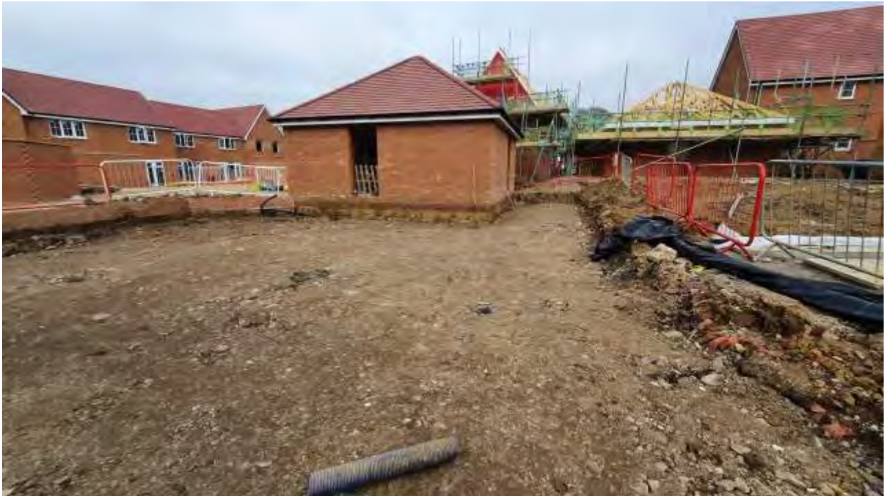
Plate 1 – View of crushed concrete installed across Plots 117-118
