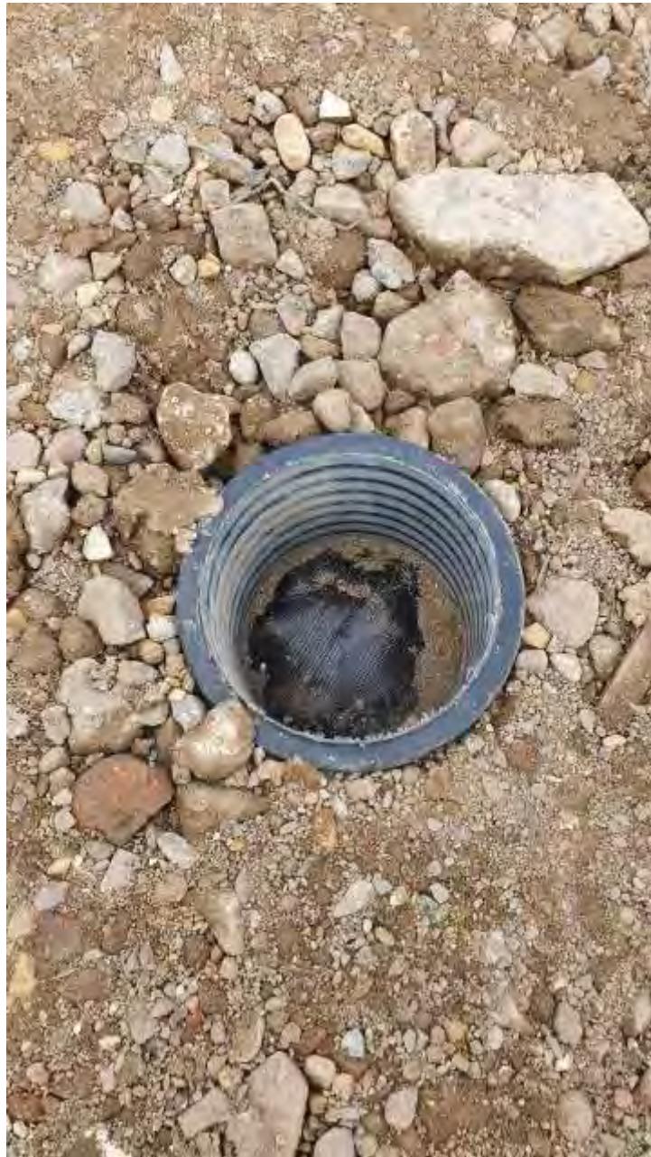
Plate 2 – View of geotextile membrane installed beneath the crushed concrete in Plot 117
