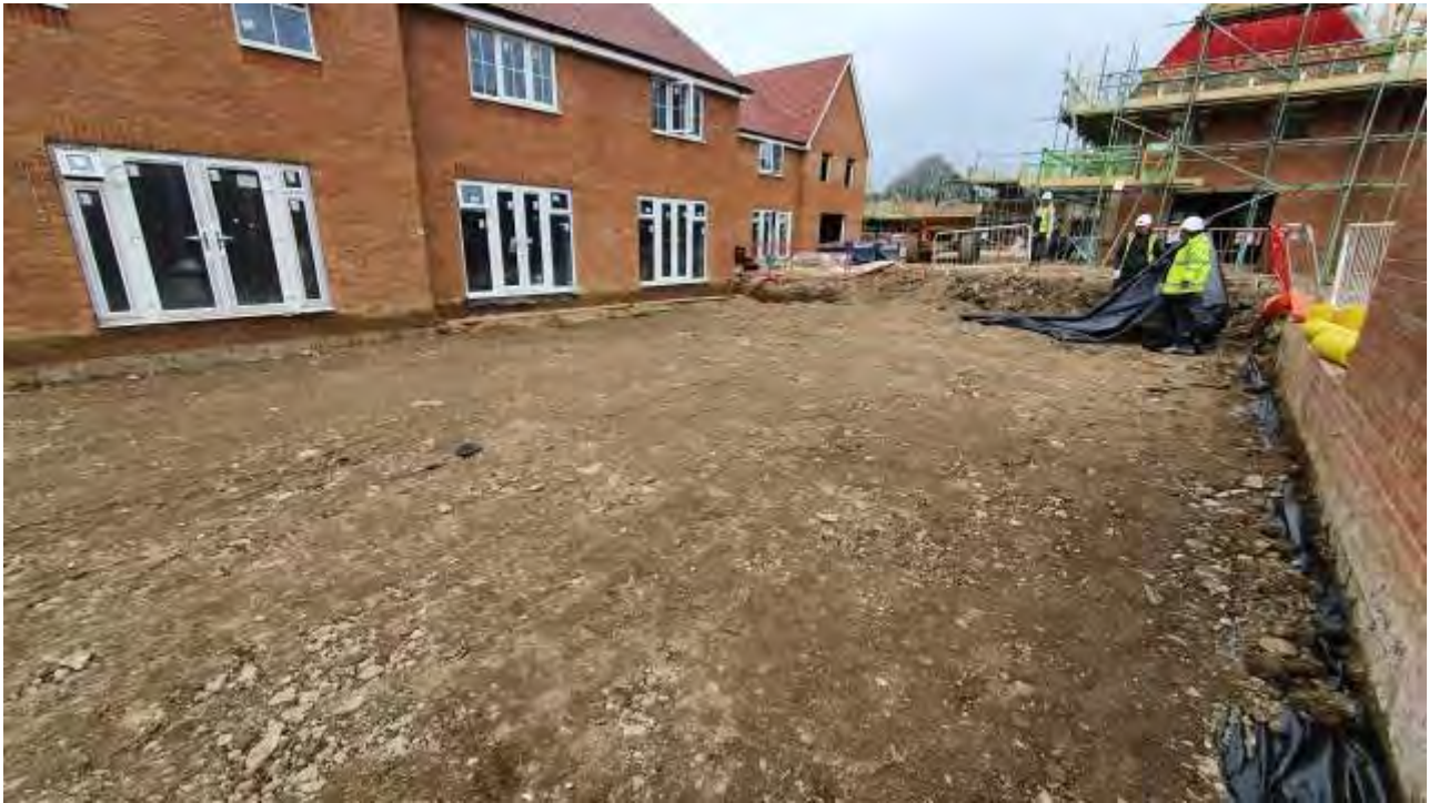
Plate 3 – Crushed concrete installed across Plots 136-138
