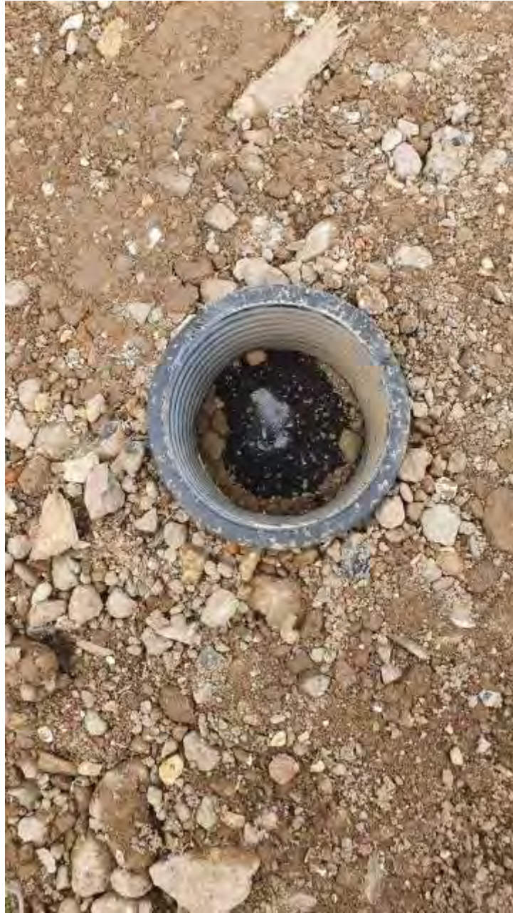
Plate 4 – Geotextile membrane installed beneath crushed concrete in Plot 136
