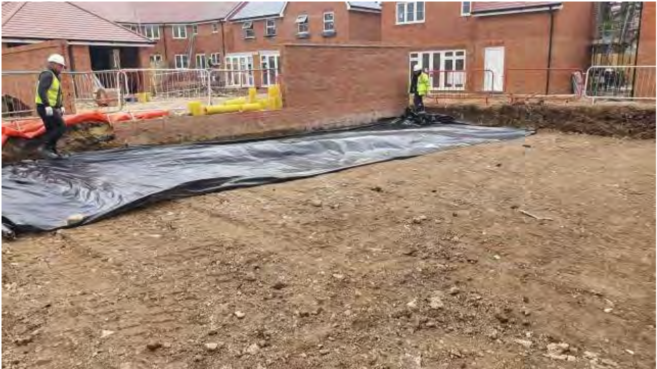
Plate 5 – View geotextile membrane being installed above crushed concrete in Plots 136-138
