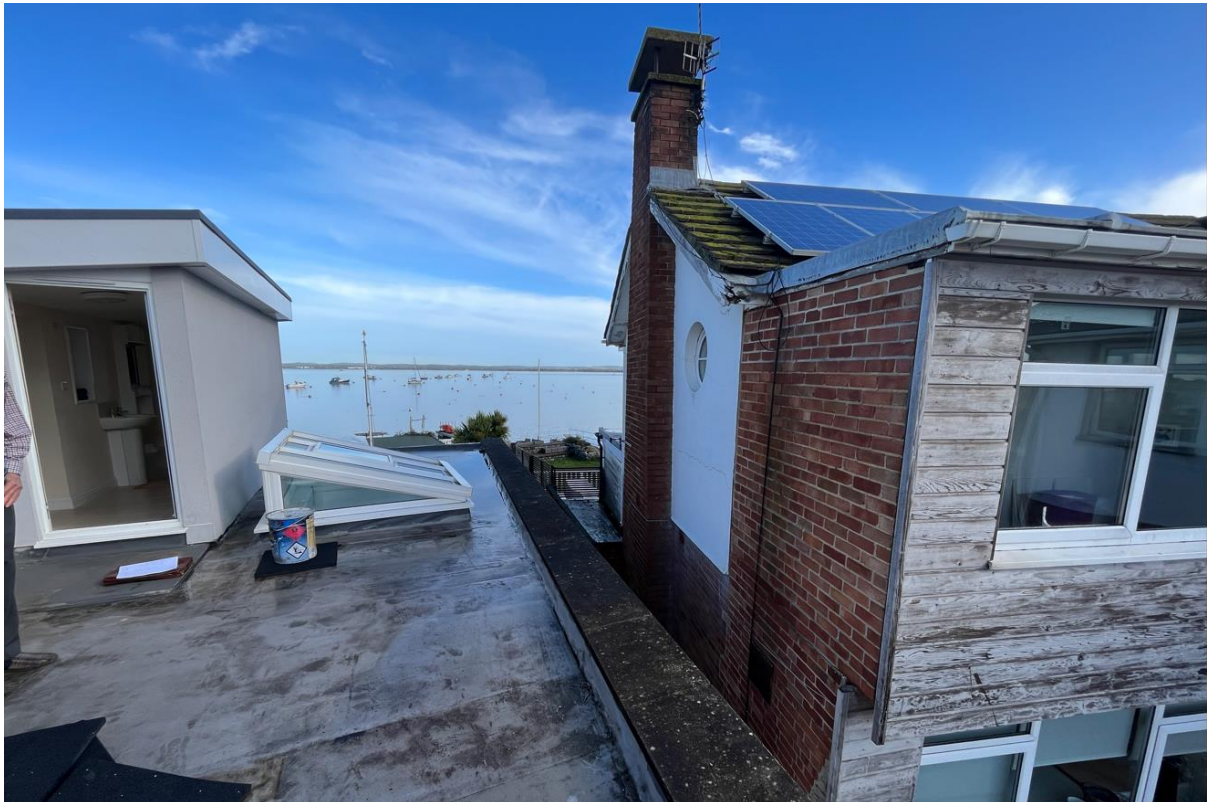
Figure 5 View Looking North between First Floor ‘Lift Addition’ & Sinah House
