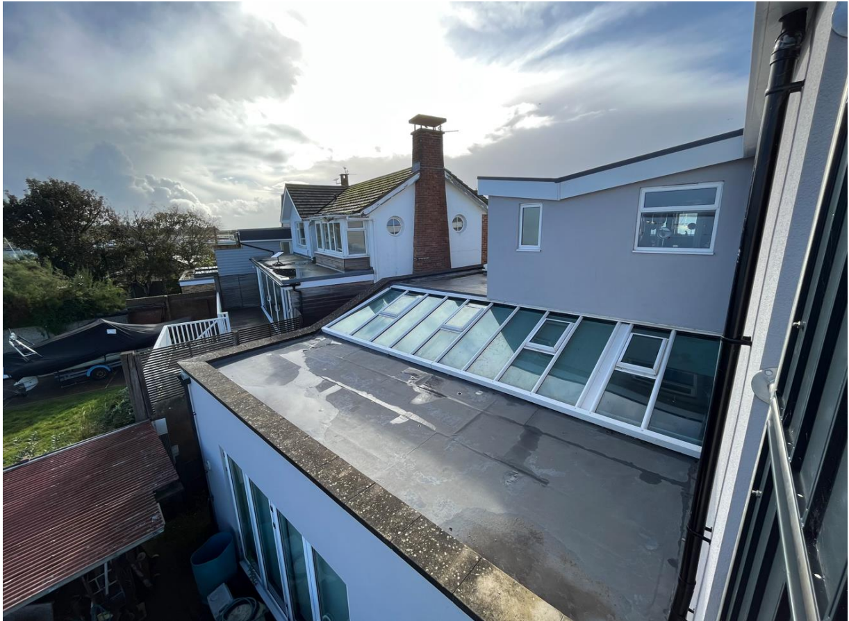
Figure 8 View from Rear First floor Balcony towards West Elevation of Sinah House
