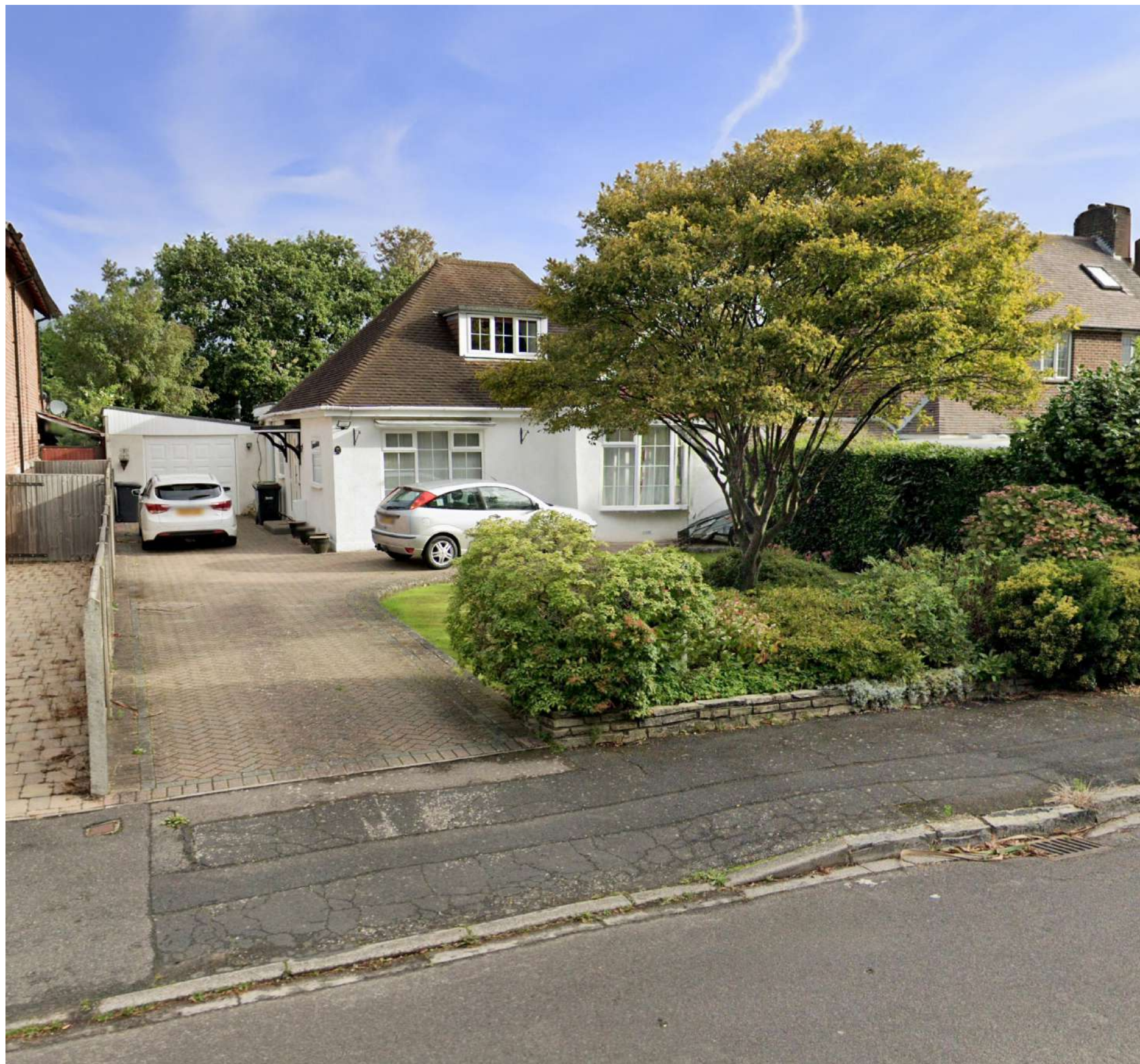
Street view of existing house.
