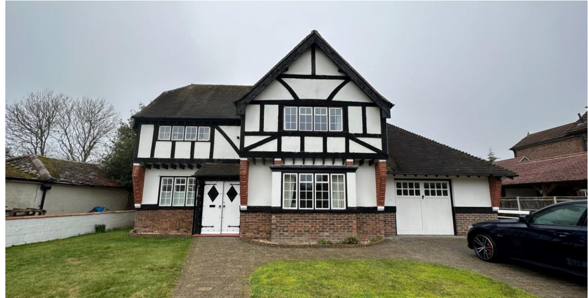
View of existing dwelling from Beach road.
