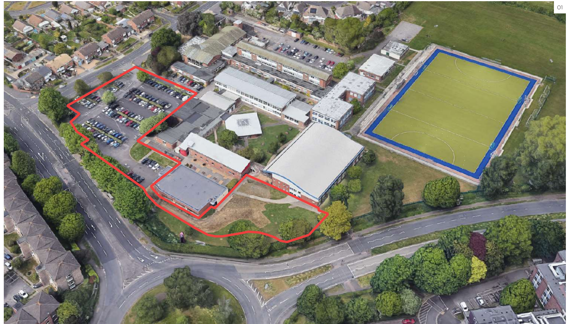
01 Aerial view of HSDC Havant Campus with the proposed development site outlined in red.
