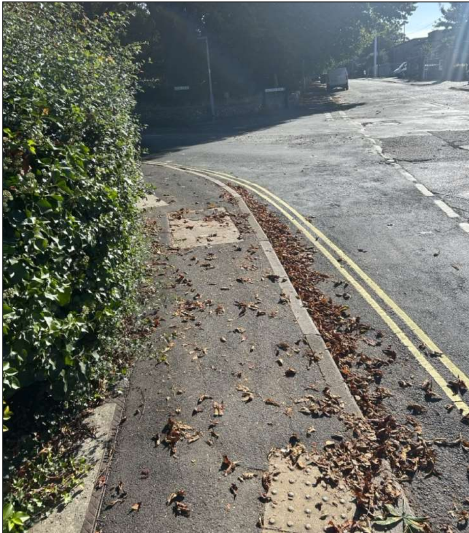
Photo 1: Lack of Visibility at the New Lane / Eastern Road Intersection
