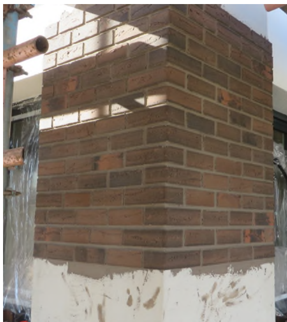
3 Brick slips being applied over external insulation
