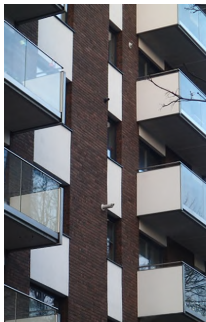
2 Finished insulated walls
