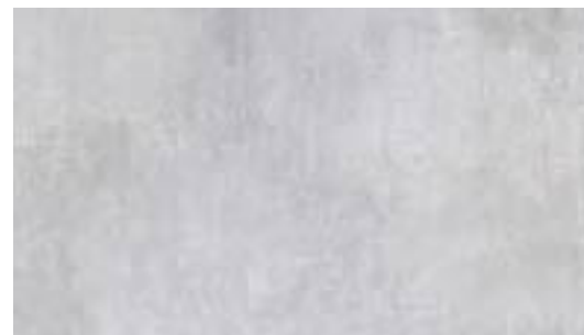
smooth concrete finish to horizontal planes
